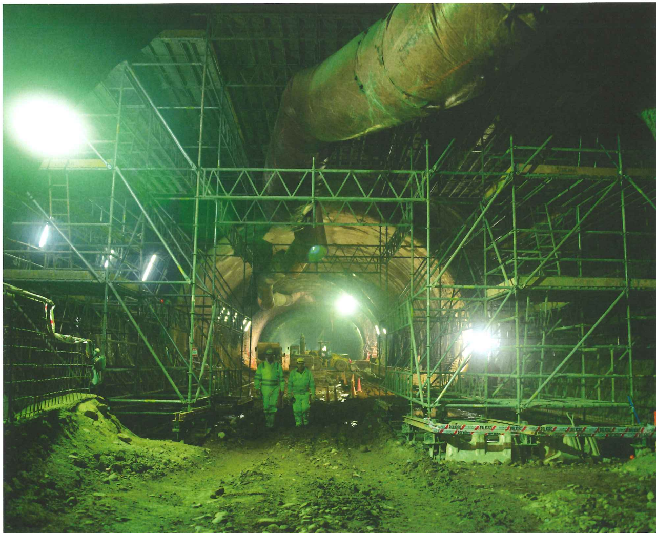
Above: NATM was used for construction of 37km of new tunnels on Santiago metro Lines 3 and 6
