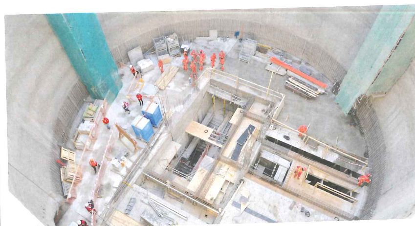
Above: View of a shaft bottom on the Santiago metro project
