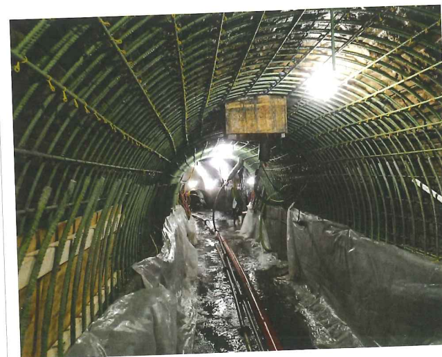
Right: A 12-inch-thick, self-supporting shotcrete overlay built inside the historic tunnel
