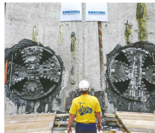
On 12 June the two Herrenknecht EPBMs broke through the target wall at the Oberhausen pumping station precisely on line and level
