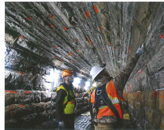
Left: Inspecting and marking the tunnel for repair work
