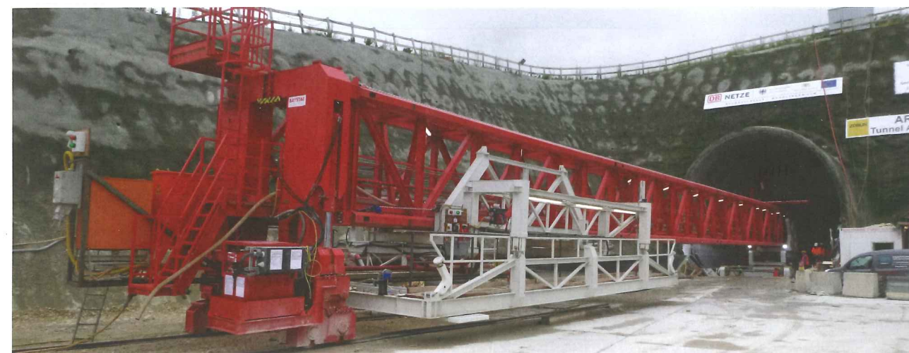
Above: Rolling formwork rig
