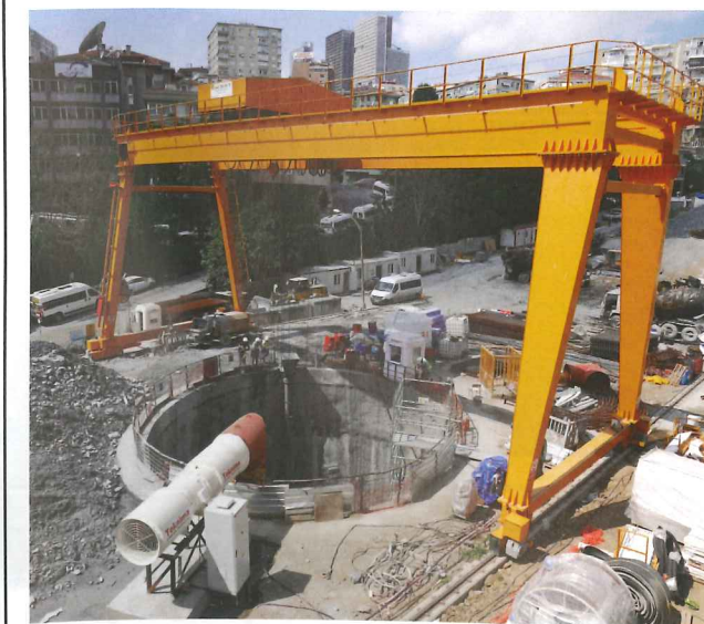
left: Launch shaft with crane for muck transport
