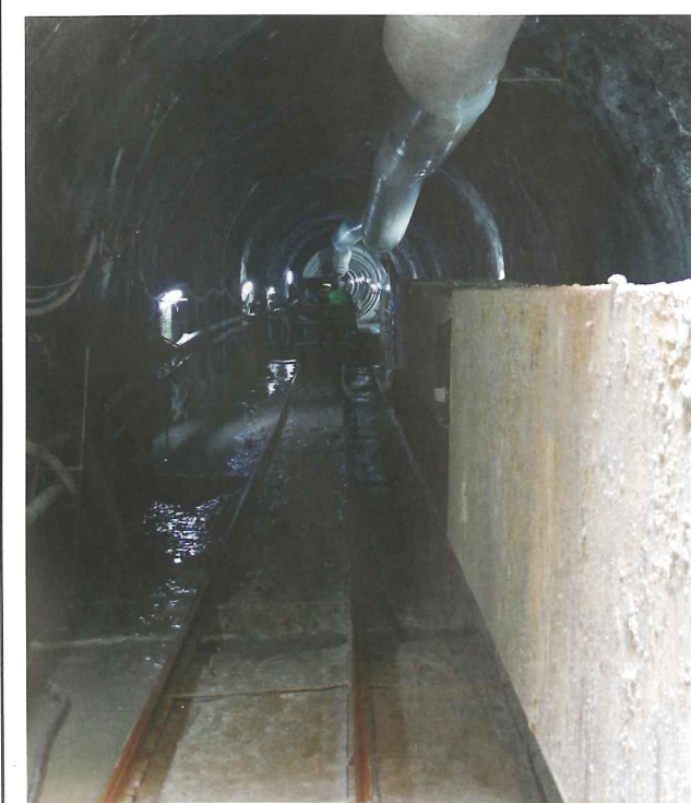
Left: Rolling stock was used to remove the muck
