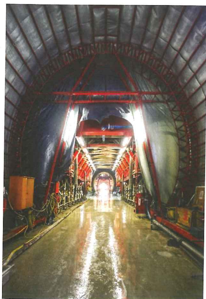
Left: Tunnel formwork rigs were supplied by Baystag
