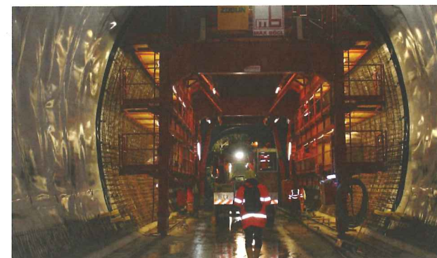
Above: Rolling formwork rig
