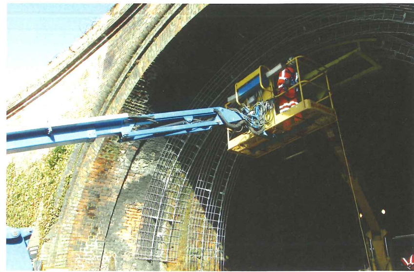
Above: Work to install RamArch at the Whiteball Tunnel
