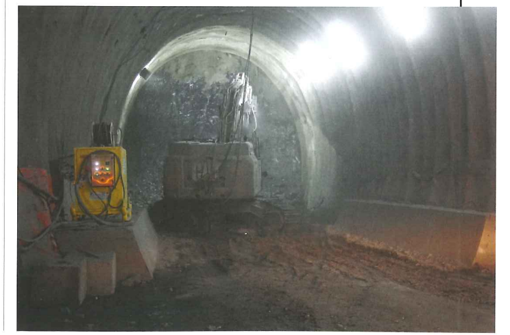
Below: 'Conventional excavation' in progress, defined by the ITA as anything non-mechanised
