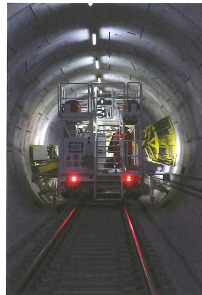
Rowa's drilling rig, page 23
