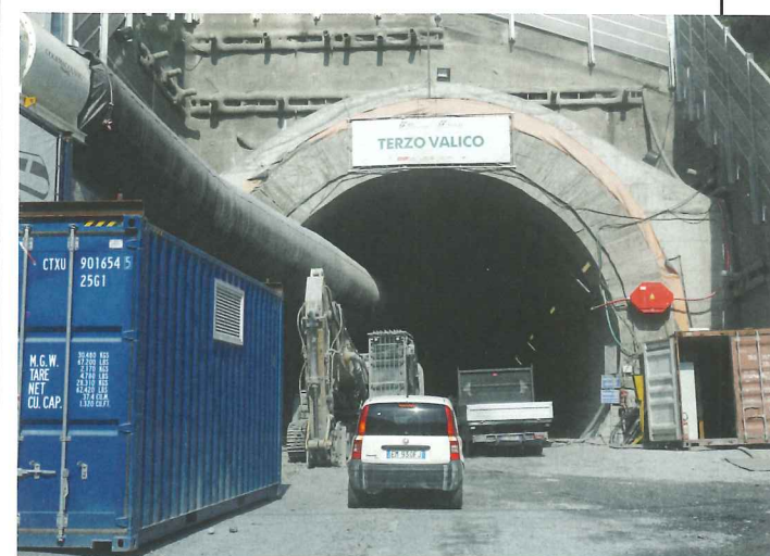
Below: View of a tunnel portal
