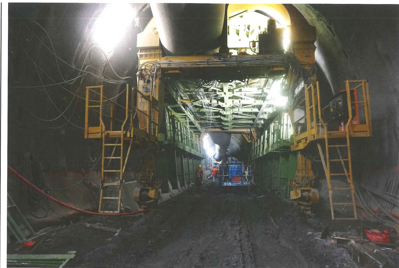
Above: Formwork in use on the project
