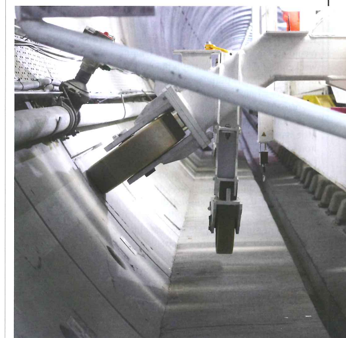
Below: The machine was bespoke for the Crossrail project
