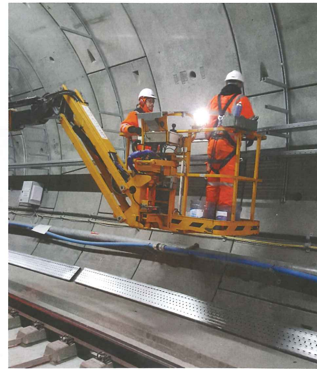
Both: Work to fit brackets to the tunnel lining
