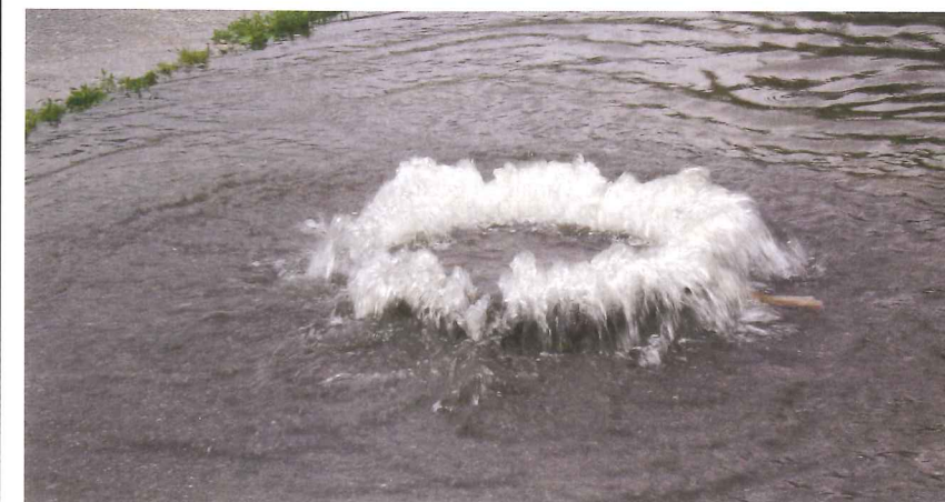
Opposite and below: Clear groundwater overflowing from a sewer onto the surrounding land
