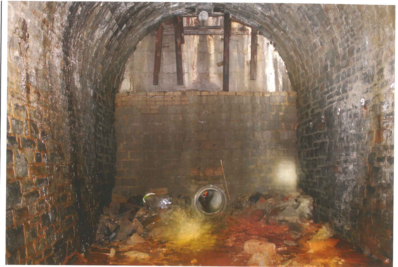
Above: The entrance pipe near the Blaencwm portal
