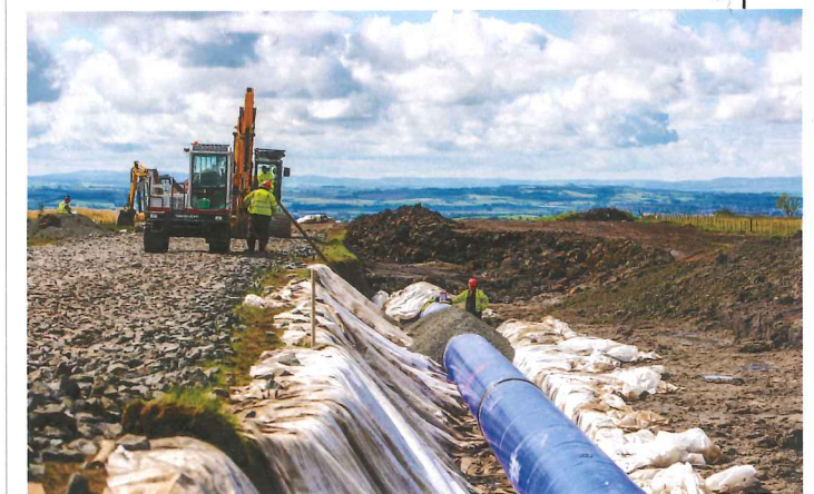
Top and centre: Herrenknecht machine preparing to pass under the rail line
