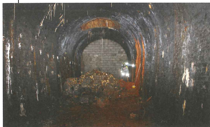
Below: Rubble at the base of the ventilation shaft is probably from a chimney above ground
