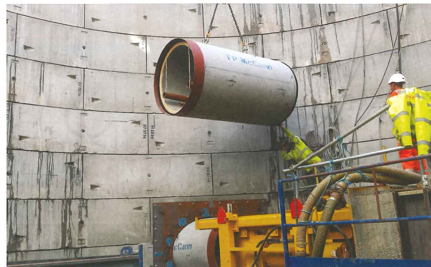
FP McCann pipes lowered down a shaft for National Grid
