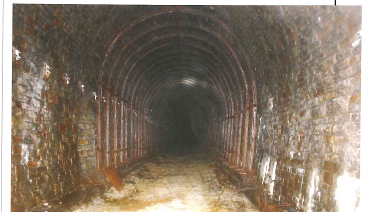
Below: The reinforcing steel ribbed section
