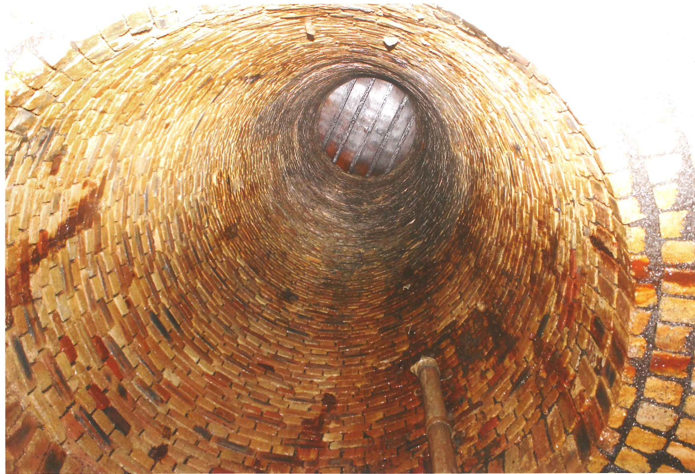
Above: The ventilation shaft is sealed at the top with a steel shutter supported by five beams
