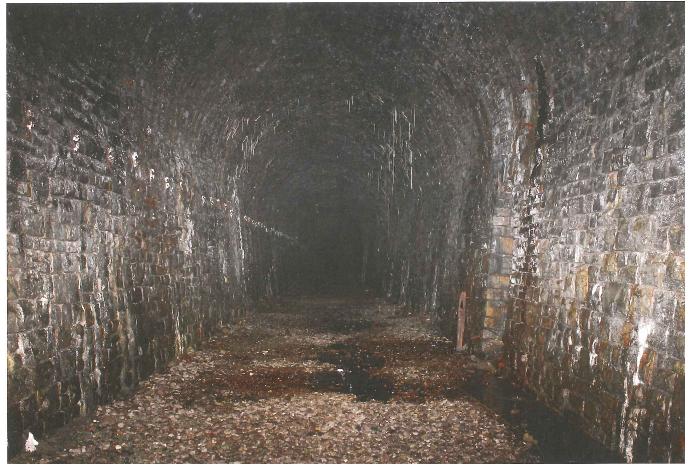
Above: A view of the masonry section of the tunnel
