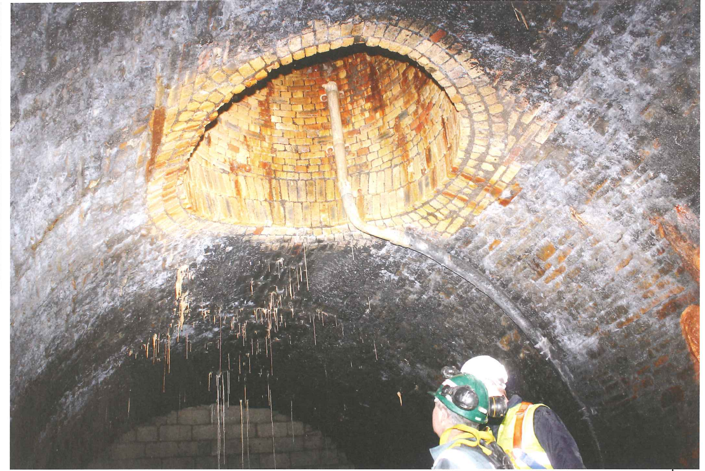
Above: Blockwork wall and ventilation shaft at the Blaengwynfi end
