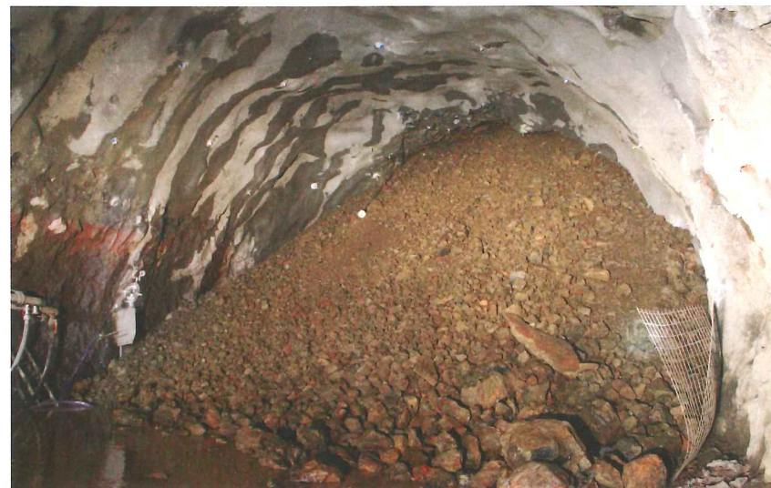
Below: Progressive collapse at the Vaðlaheiði tunnel
