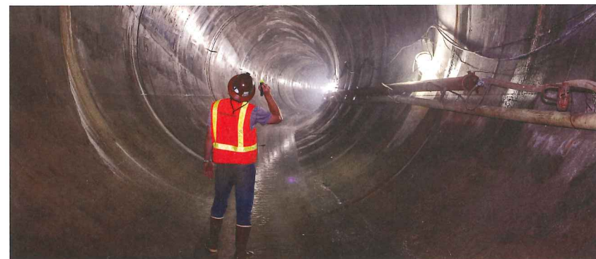
Continuous conveyors will navigate curves as sharp as 300m along the route
