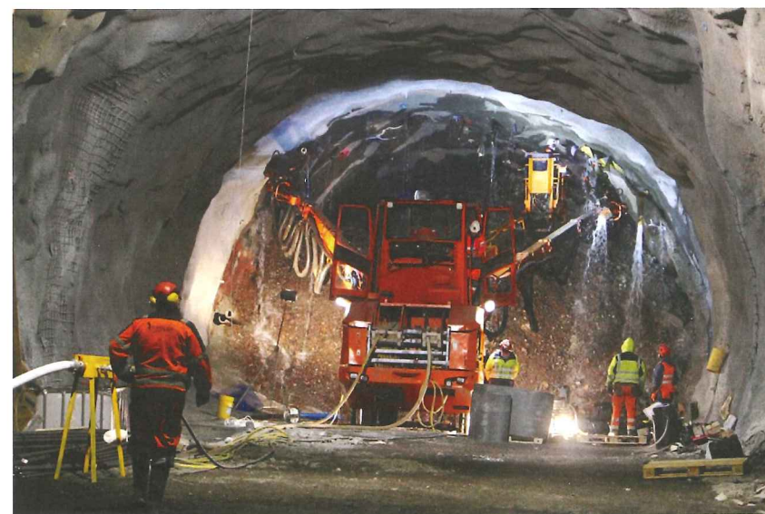
Below: Fnjosk consolidation grouting
