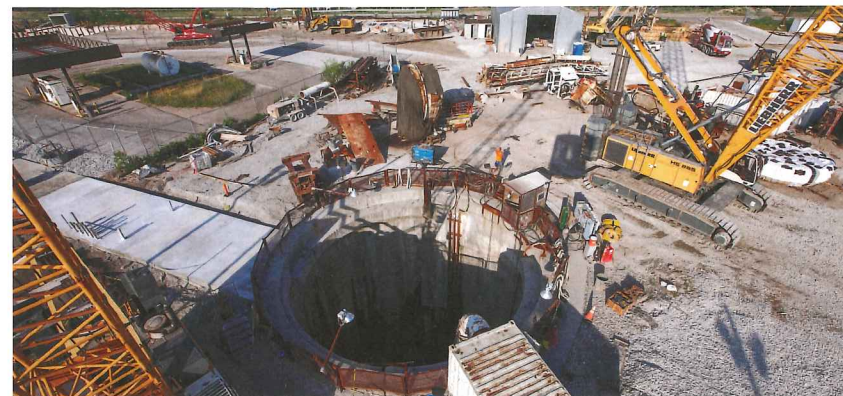
The TBM was launched from the 67m-deep White River shaft
