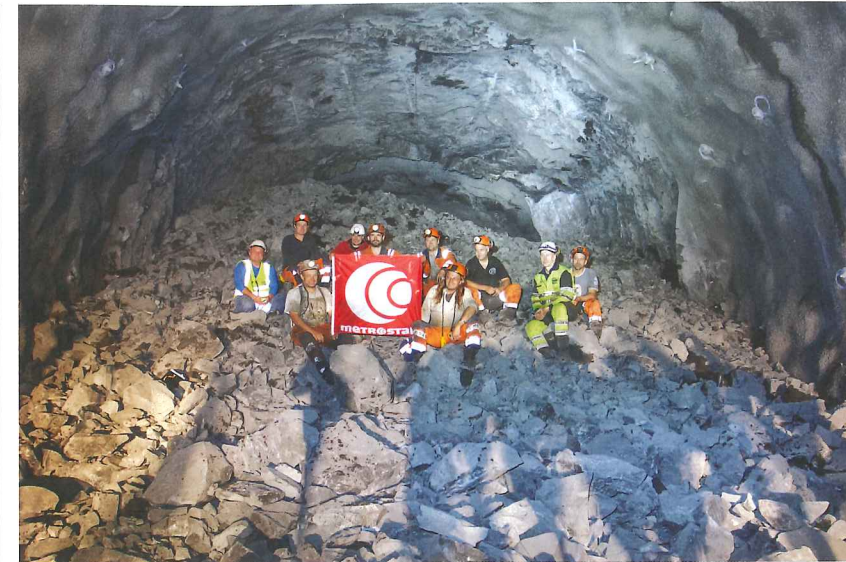
Breakthrough at Nordfjordur in September 2015
