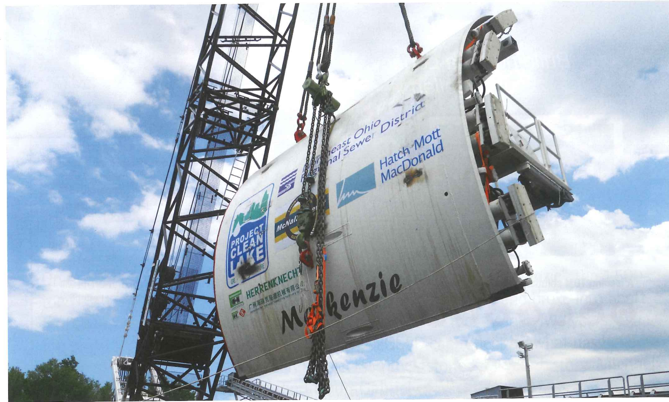
Top: Main tunnelling shield at work on the project
