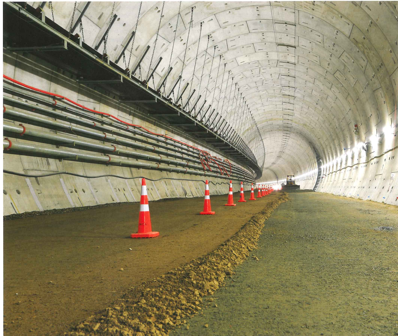
Above: Road surface preparatory works
