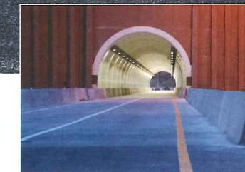
Carlin Tunnel Nevada, USA First highway rated speed tunnel fully lit with LEDs in North America
