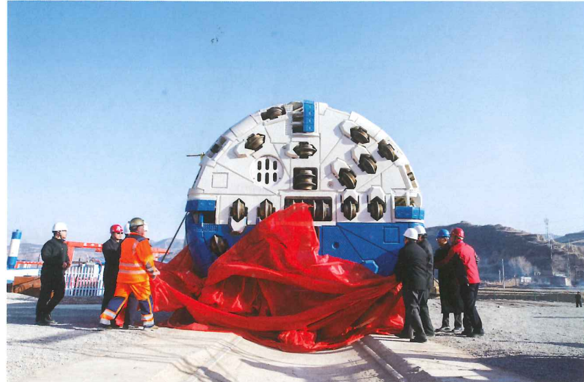
Top: Hexagonal segments are manufactured and stored at the large T1 jobsite
