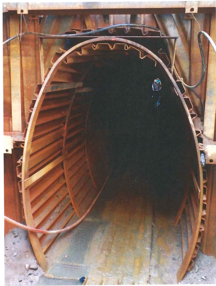
Above: View of the shaft-tunnel interface on the interceptor sewer in Benesov
