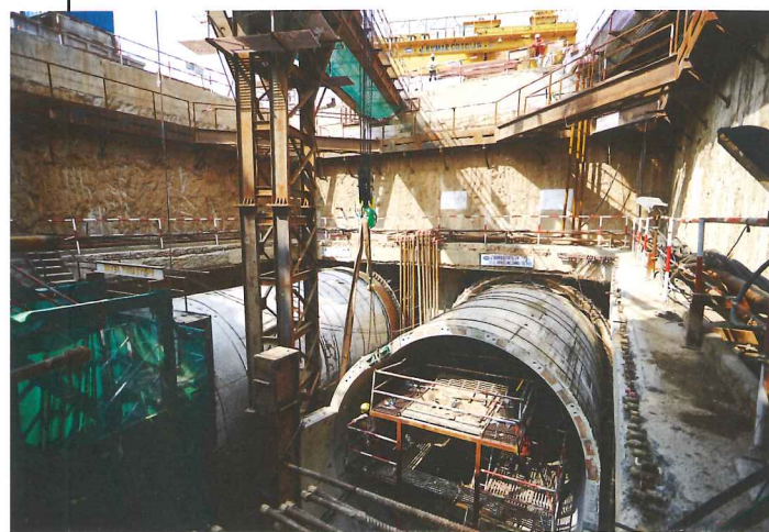
Below: CC20 work well under way after initial land acquisition issues
