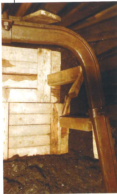
Left: Face timbering within highly weathered rock (Interceptor Sewer 'H' in Prague)
