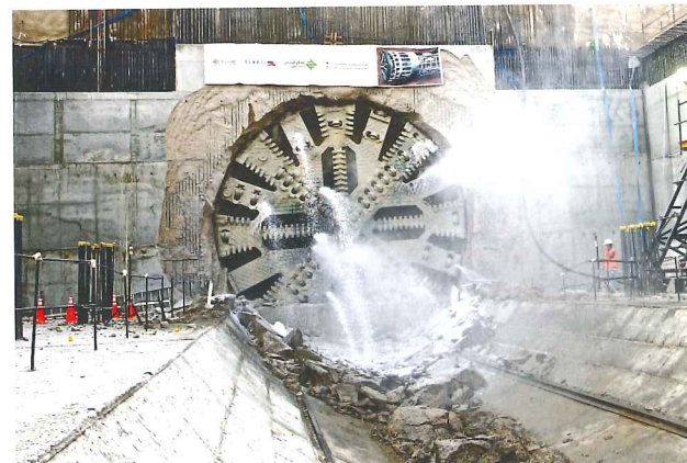
Breakthrough on the first stretch of tunnel
