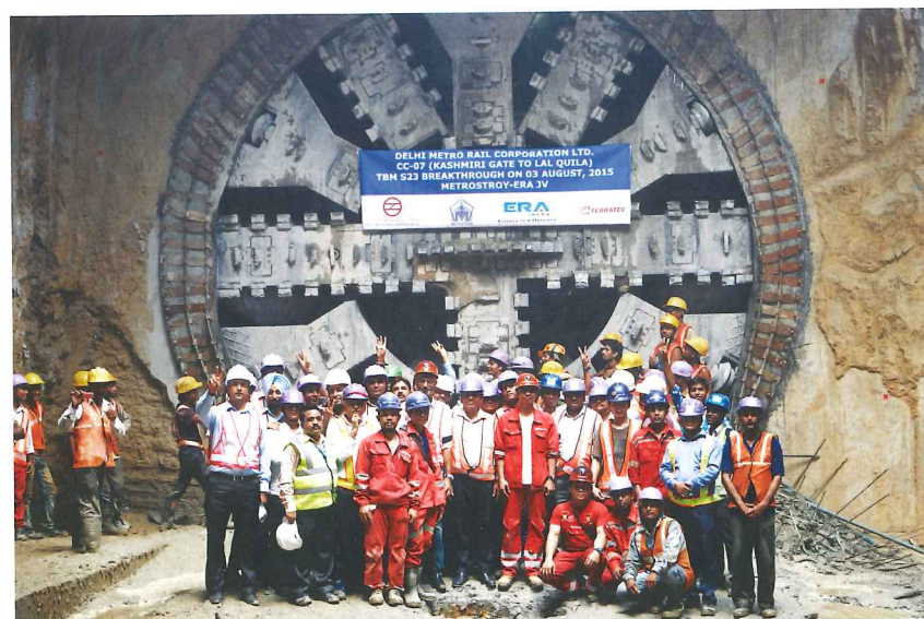
Breakthrough was achieved at the Delhi Metro CC-07 reception shaft
