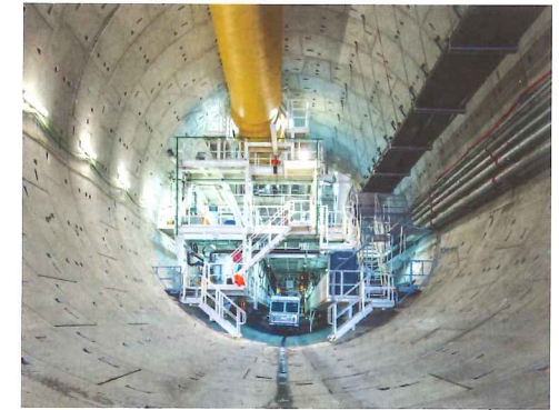
Alice is the largest TBM ever used in the southern hemisphere
