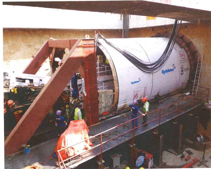
Below: TBM preparing to launch off a frame
