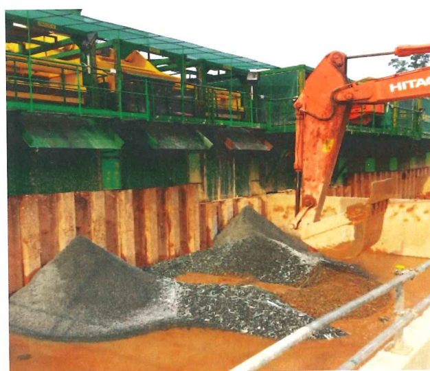
Below: Tagore site STP spoil pit showing initial excavation after tunnelling through fibre-glass reinforced piled wall
