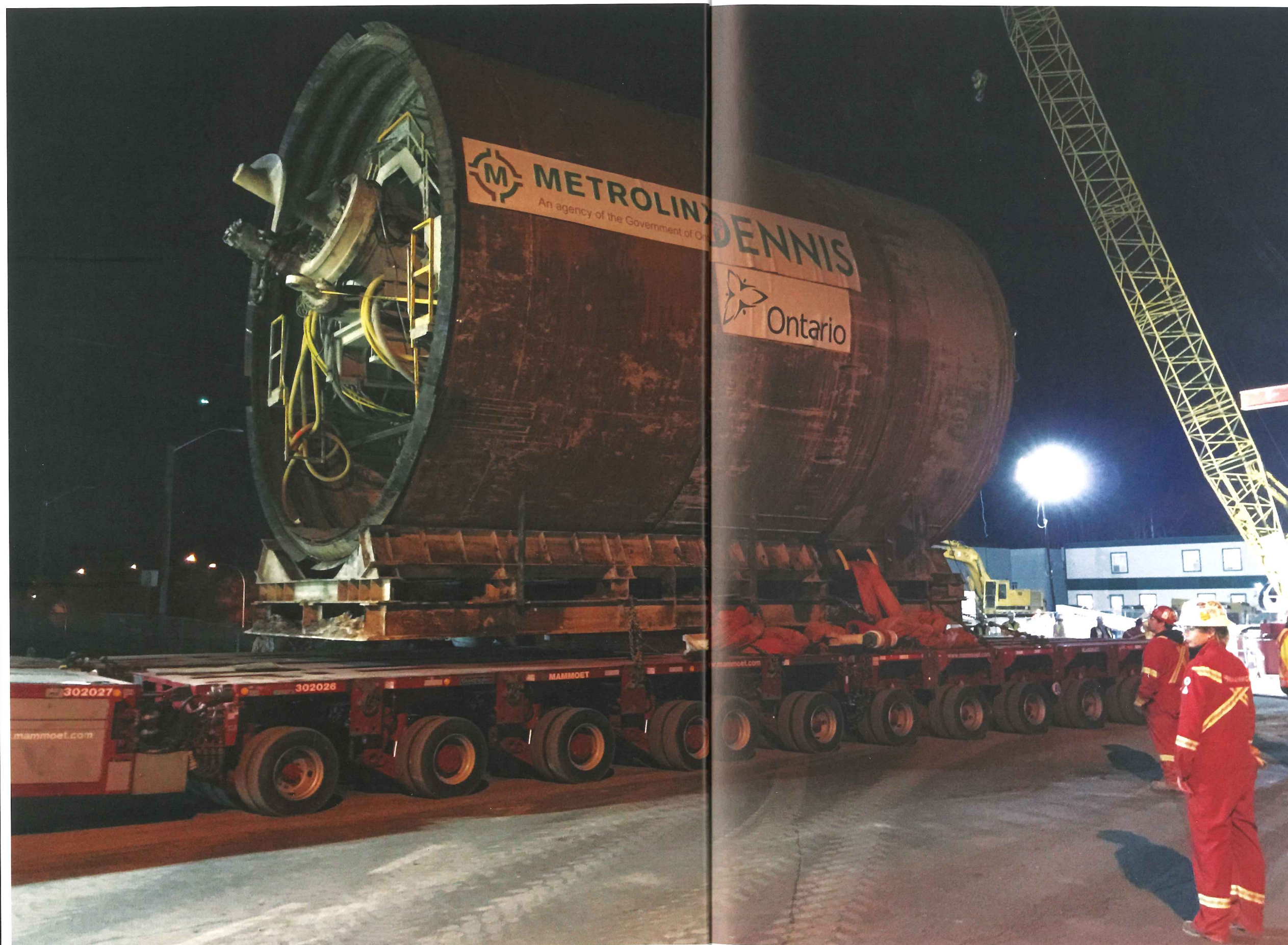
Left: Over the weekend of April 17-20, in the early morning hours, Crosstown Transit Constructors, a joint venture of Obayashi Canada, Kenny Construction, Kenaidan Contracting and Technicore Underground, extracted the two TBMs that have been tunnelling the western segment of Toronto's Crosstown's underground section, from a shaft located just west of Allen Road.
