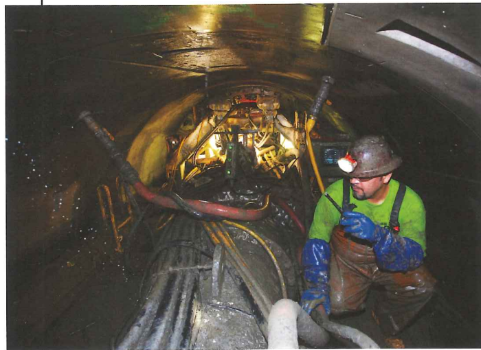
Above: A crew member inspects the TBM
