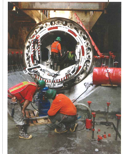
Right: The 3.8m EPBM, manufactured by Caterpillar, was launched in August 2012
