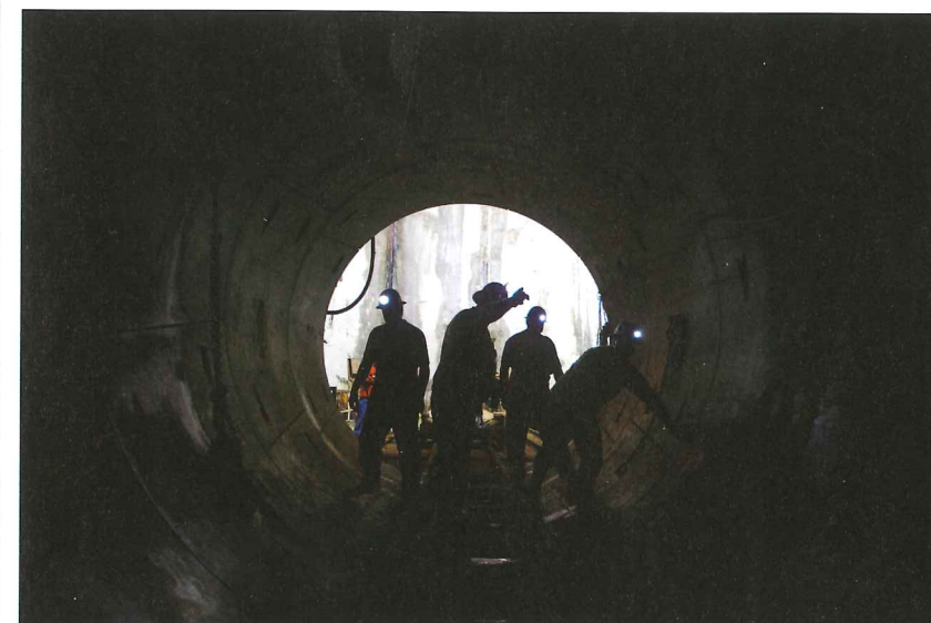
Below: Completed tunnel before installing the welded steel pipeline
