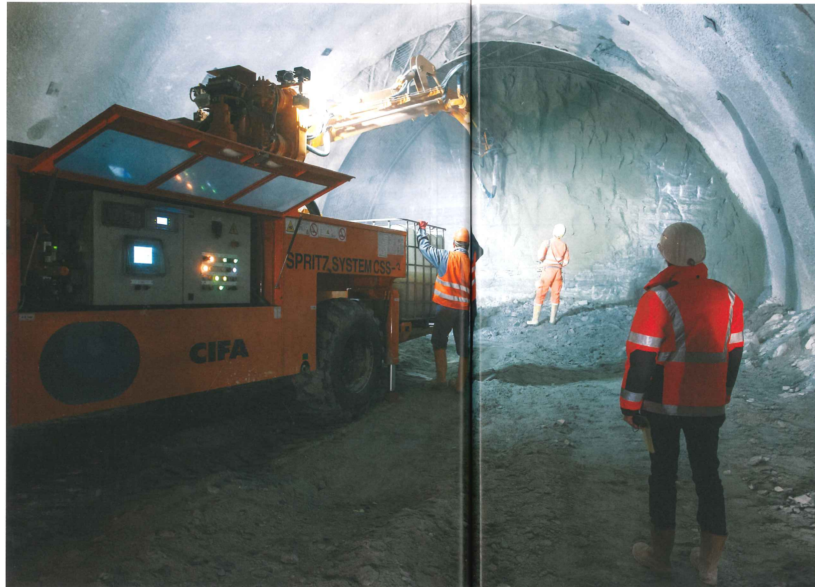
Above: Cifa Spritz System in operation at Brenner
