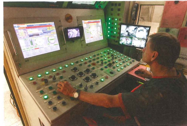
Seattle LRT TBM operator's cabin
