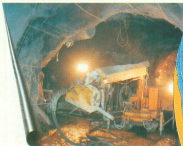
El Indio, Chile Small spraying system SIKA powder accelerator
