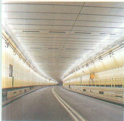
Callahan Tunnel, Boston, MA
