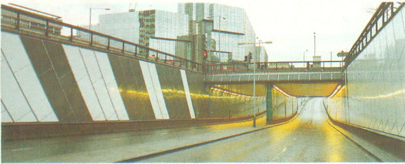
Euston Road Underpass, London, UK
