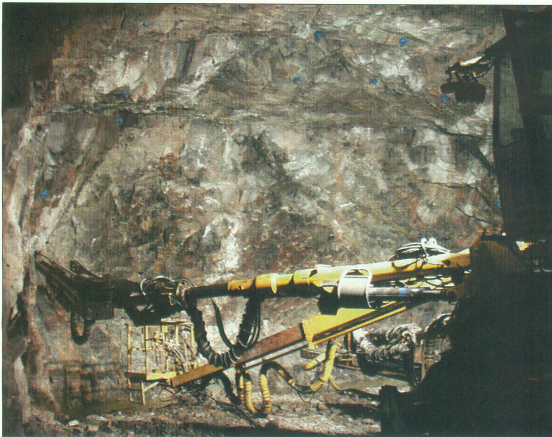
The Atlas Copco computer assisted Rocket Boomer 353S drilling jumbo at work on the Frøya Tunnel
