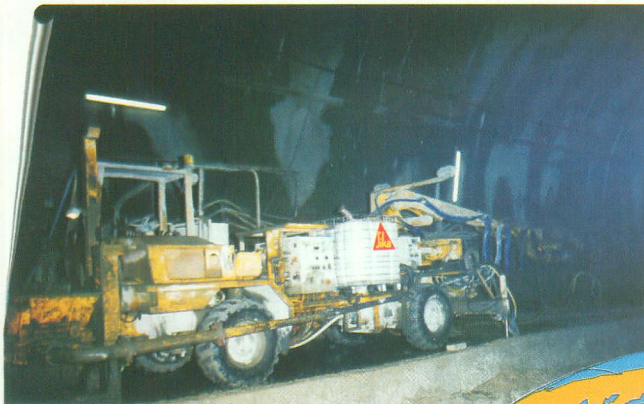
ICE, Germany Spraying system with pump and alkali free accelerator
