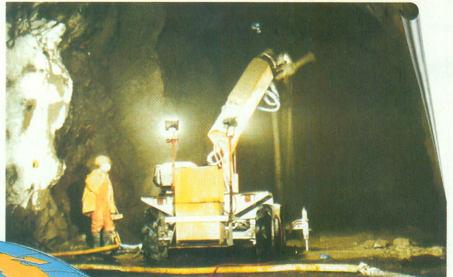
Neat, Switzerland Spraying boom, Rotor machine and pump SIKA accelerator, plasticizer
