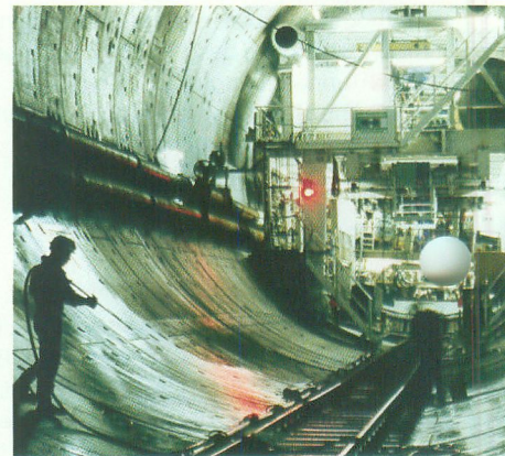
High-tech tunnelling deep under the busy river Elbe
