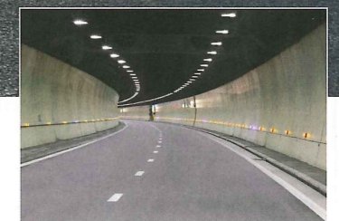
Chamoise tunnel, France Fully lit with LEDs
