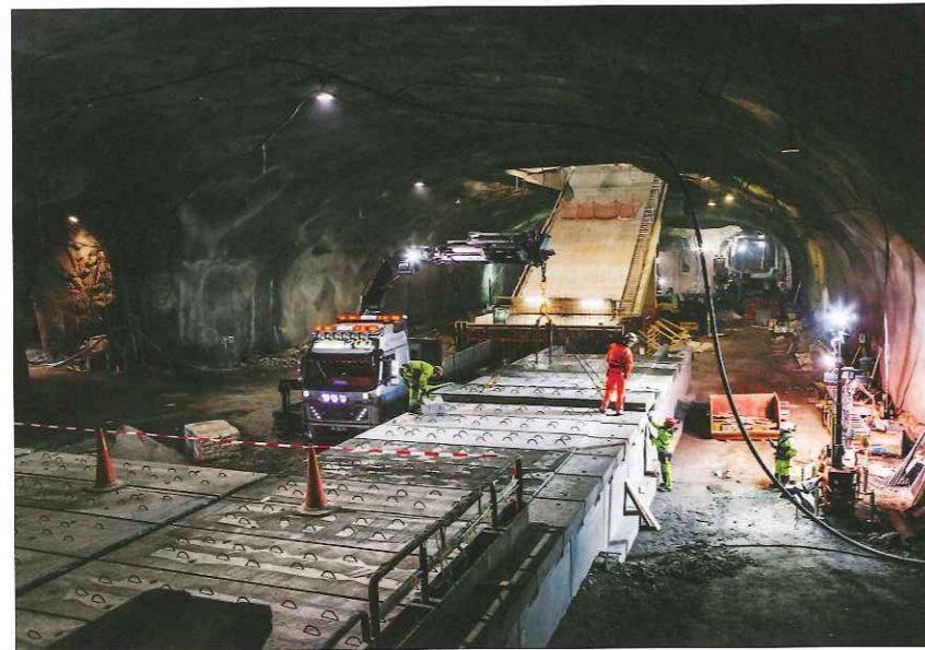
Above: Escalator shaft at the Stockholm City station, December 2013 MIKAEL ULLÉN
