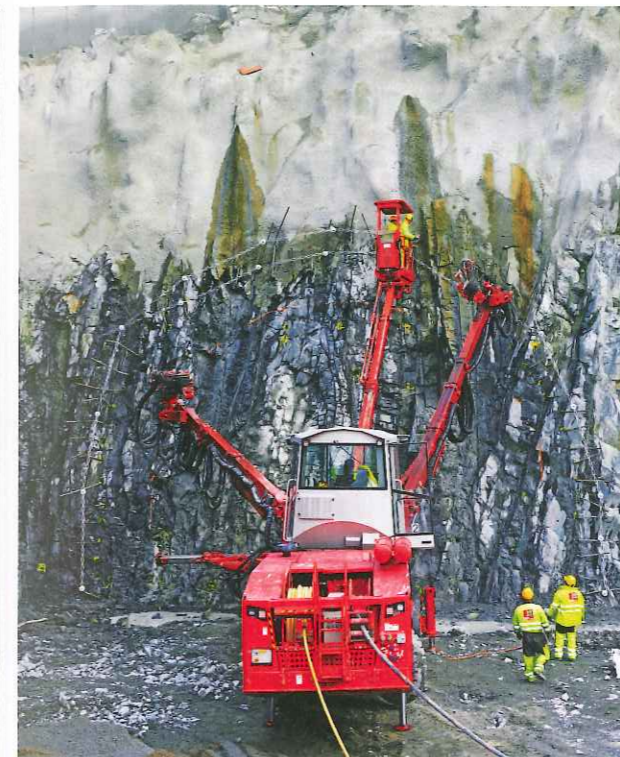
Above: Preparing to blast at Solbakk for Ryfylke Tunnel
