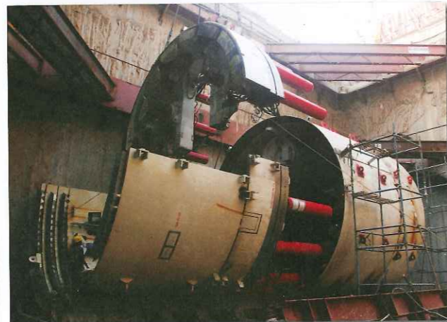
All: TBM assembly at the shaft bottom in Delhi
