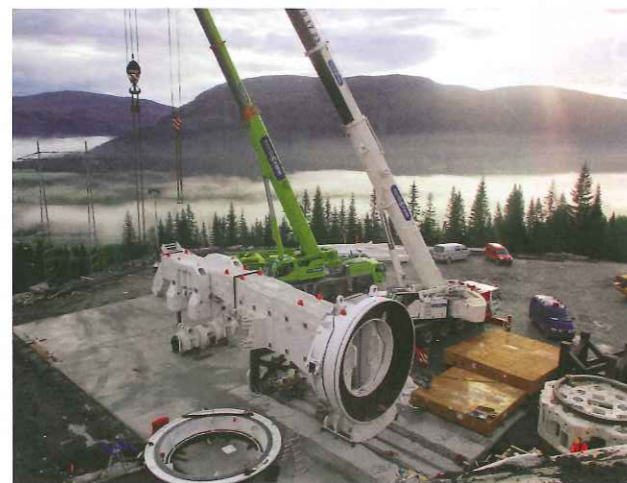
Assembly of the Robbins TBM in Norway
