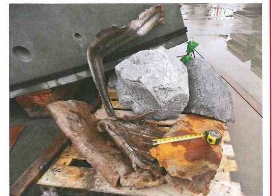
Pieces of the steel pipe, image courtesy of WSDOT
