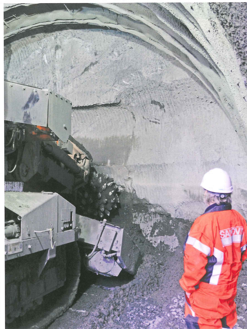
Below: A Sandvik engineer oversees excavation
