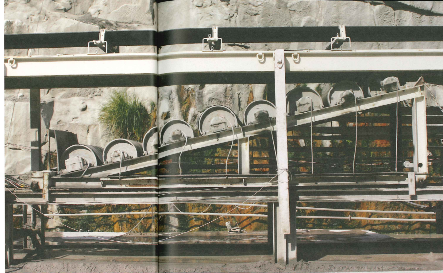
Left: The continuous conveyor system carries muck from the TBM
