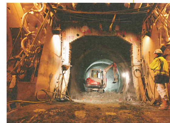
Right: Excavating a cross-passage in frozen ground; Right, bottom: Installing cross-passage concrete reinforcement cage within a waterproofing membrane layer
