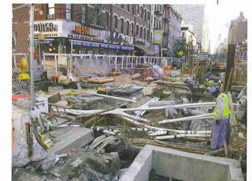
Below: Utility work along Second Avenue
