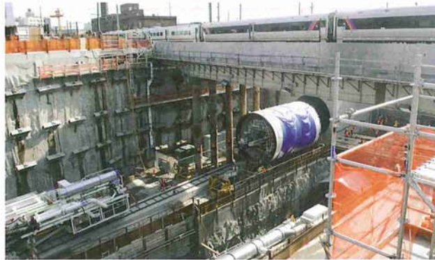
Above: Construction was scheduled to begin in April
