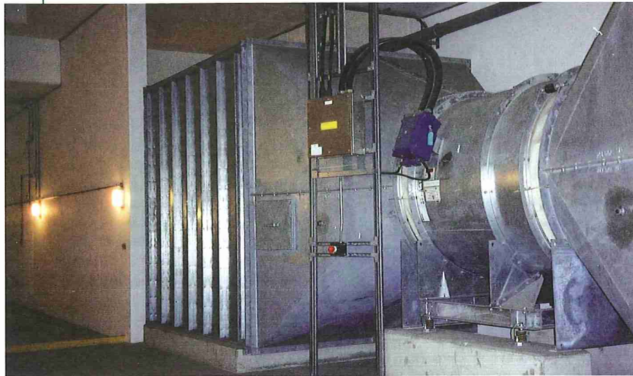
Above: Modern fan room with axial fans (300m 3 /s in total) and sound attenuators (Photo: Dr Sean Siew)
