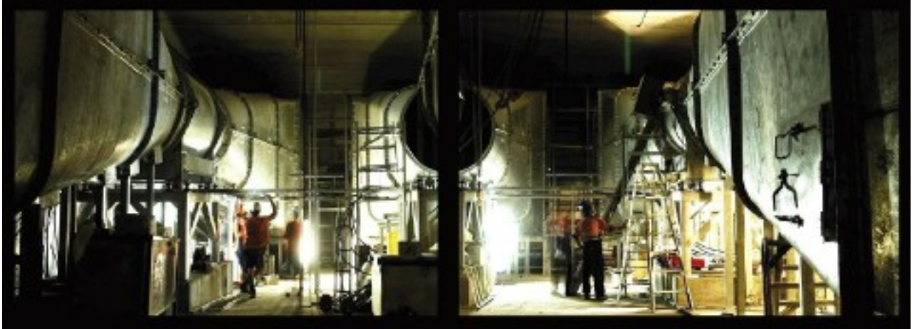
Above: Modern fan room with axial fans (300m 3 /s in total) and sound attenuators (Photo: Dr Sean Siew)
