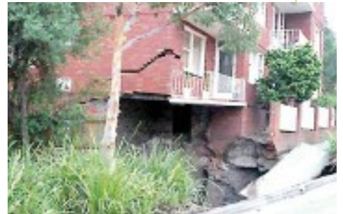
Above: The corner of the residential building directly over the collapse; Left: Plan diagram of the Lane Cove tunnel project with the collapse site shown
