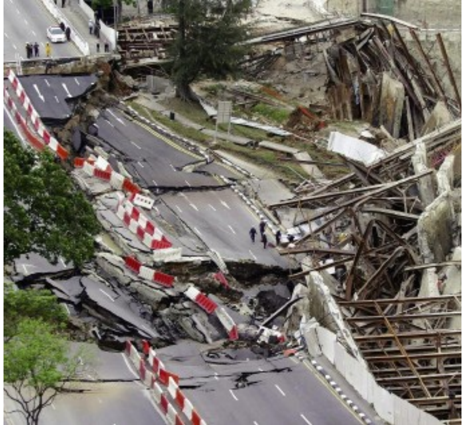
Above: The Nicoll Highway collapse of 2004
