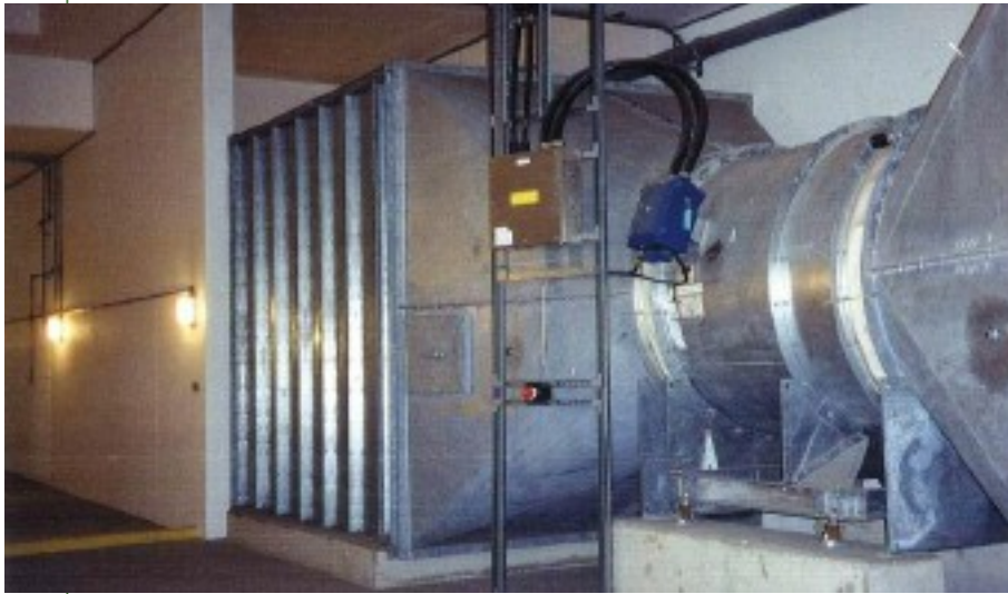
Above: Modern fan room with axial fans (300m 3 /s in total) and sound attenuators (Photo: Dr Sean Siew)
