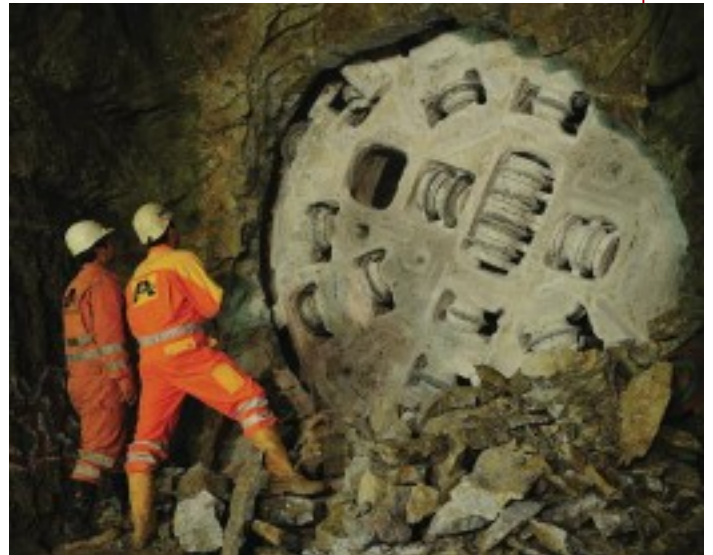
Above: China's Pinglu Tunnel saw a breakthrough in late 2010
