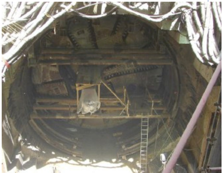
Above: Reaching the buried TBM from the rescue shaft; Below: The recovery works advance at the TBM
