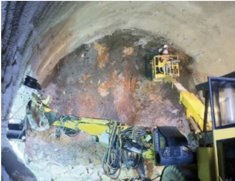
Above, left: Excavation and support inspection in Tunnel 3A Above, right: Excavation in an Anabe tunnel during an earlier stage of fast rail link construction
