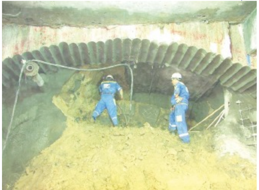
Above: Reaching the buried TBM from the rescue shaft; Below: The recovery works advance at the TBM
