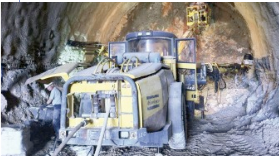
Below: Drill and blast work underway in Tunnel 3A
