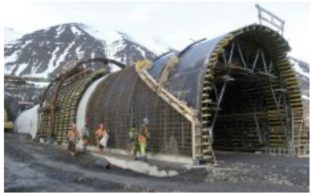
Above: The horseshoe-shaped gantry crane running on tracks was used to lift reinforcement into place for the next stage of portal construction
