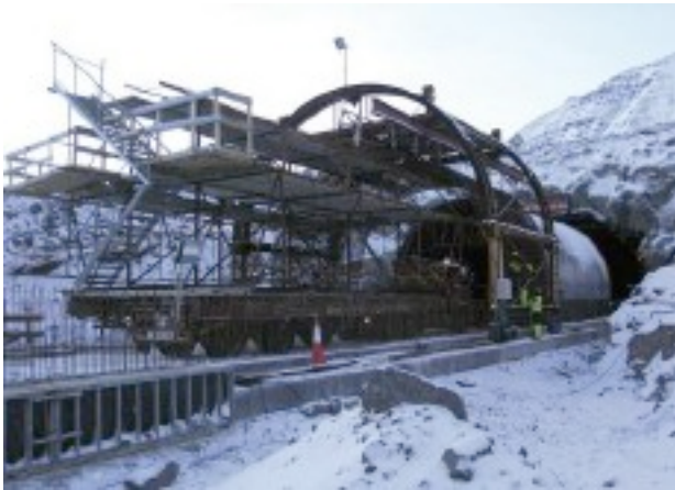
Above: The horseshoe-shaped gantry crane running on tracks was used to lift reinforcement into place for the next stage of portal construction
