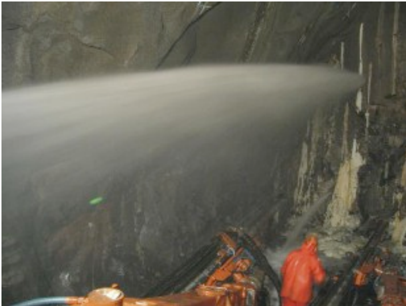
Left: Cold, high-pressure water was frequently encountered during tunnelling
