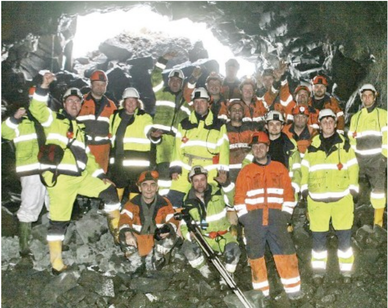
Above: A well earned celebration at Siglu on holing through, in March 2008, to Hedinsfjordur valley between the tunnels under construction
