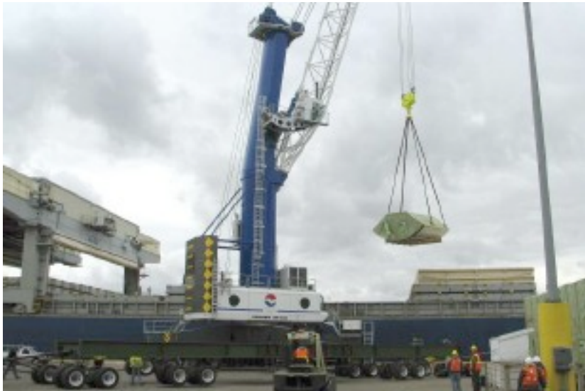
Above: The new Liebherr heavy lift cranes have a 140t capacity
