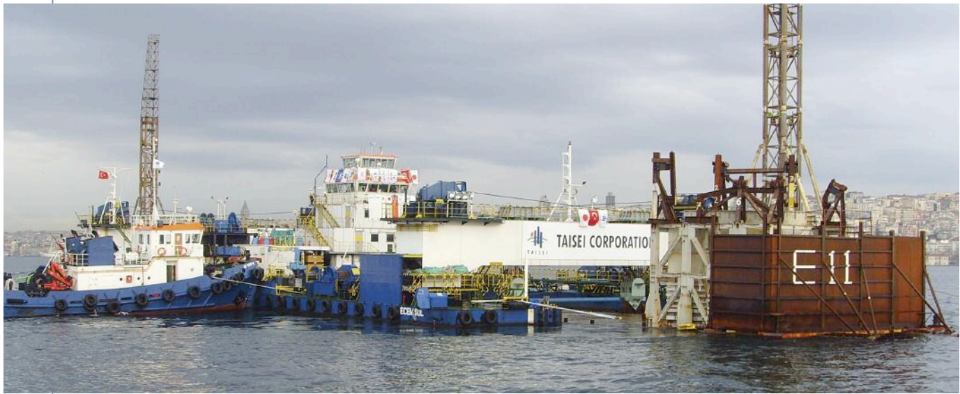
Above: Element E11 is immersed by ballasting 3 per cent of the tube's weight Left: Backfill is added for protection and to return the seabed to its original profile
