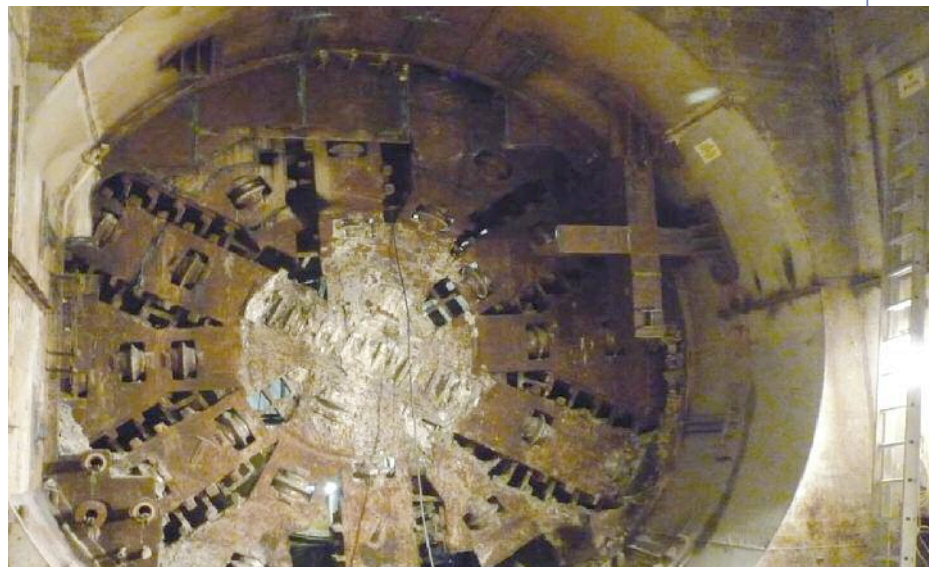
Below: TBM 4 breaks through at immersed tube element E11
