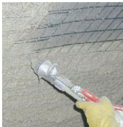
Far left: Mesh is fixed to the main lining with 'pig tail' anchors before applying FireBarrier 135
