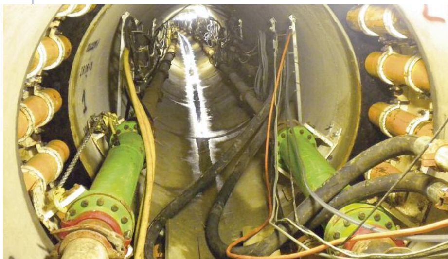
Below: Intermediate jacking points are placed every 140m along the drives
