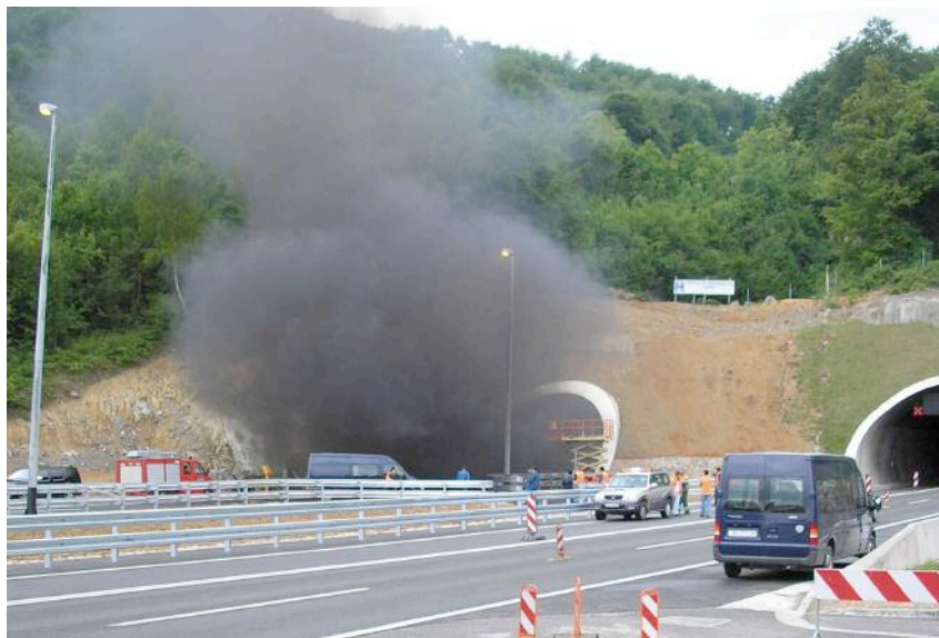
Left, top: Smoke emerging from the Veliki Glozac Tunnel in Croatia during testing of Lios Technology's fibre-optic linear heat detection system
