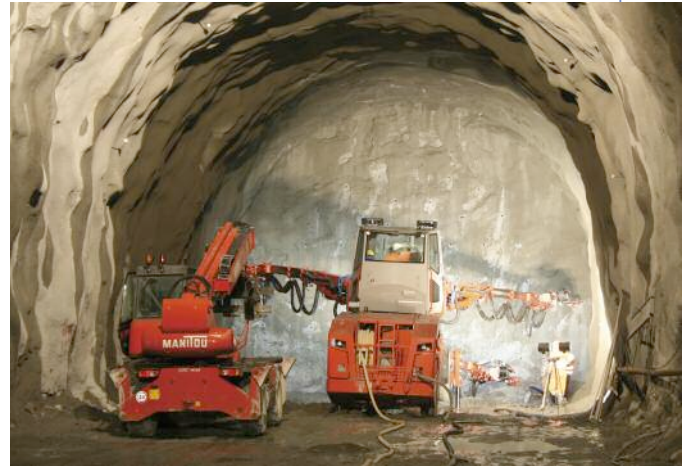
Above: Excavation of an exploratory tunnel prior to the main Brenner Base tunnels
