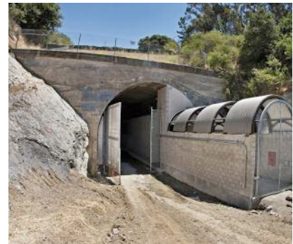
Top: The rail compartment of the Cal Park Tunnel showing sprayed concrete sidewall support and the concrete masonry divider to the pedestrian side (right) [Photo: Jacobs Associates – Sue Bednarz]; Above, left: Looking south through the completed multi-use pathway passage [Photo: Jacobs Associates – Sue Bednarz]; Above, right: Cal Park Tunnel south portal showing multi-use pathway transition structure [Photo: Jacobs Associates – Sue Bednarz]
