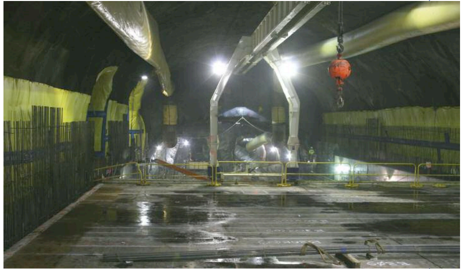
Above: Formwork at the 34th Street Station's mezzanine, looking south
