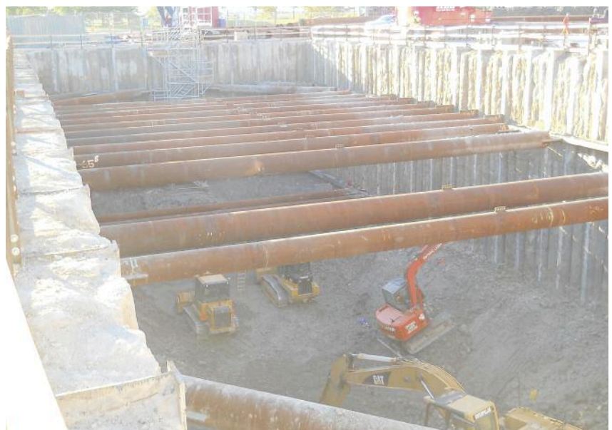
Above: Construction is set for completion in 2014
