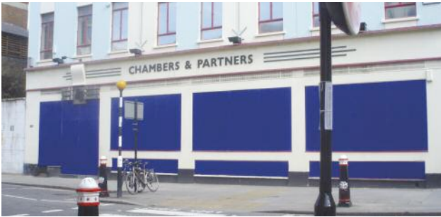
Left: The Lindsey Street properties have now been secured for demolition
