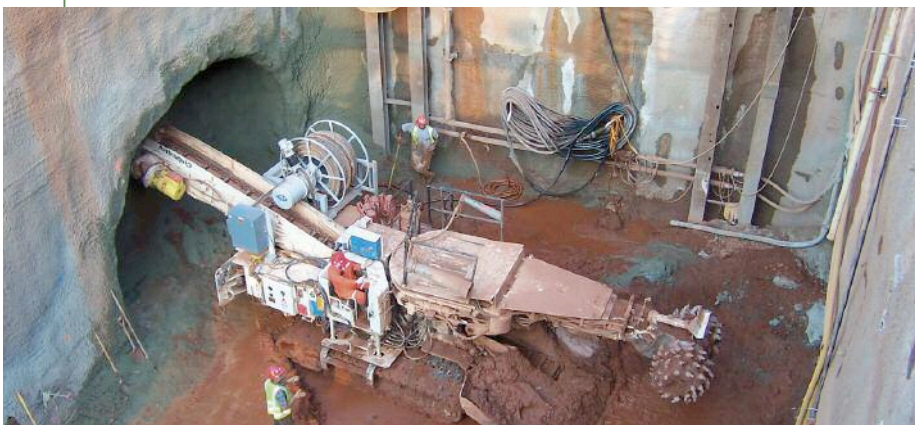
Left: An AM75 roadheader rebuilt by Antraquip for work on the Washington Dulles Airport West APM tunnel
