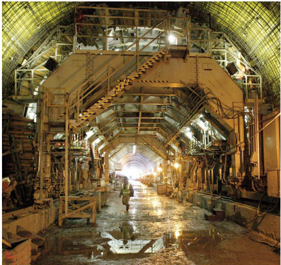
Above: Permanent lining installation in progress viewed from the Ceresola reinforcement gantry end (Photo: John Huseby, Caltrans Photographic Dept)
