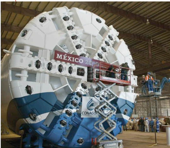
Left: The three EPBs are being assembled in Corpus Christie
