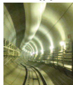
Heathrow Baggage Tunnel
