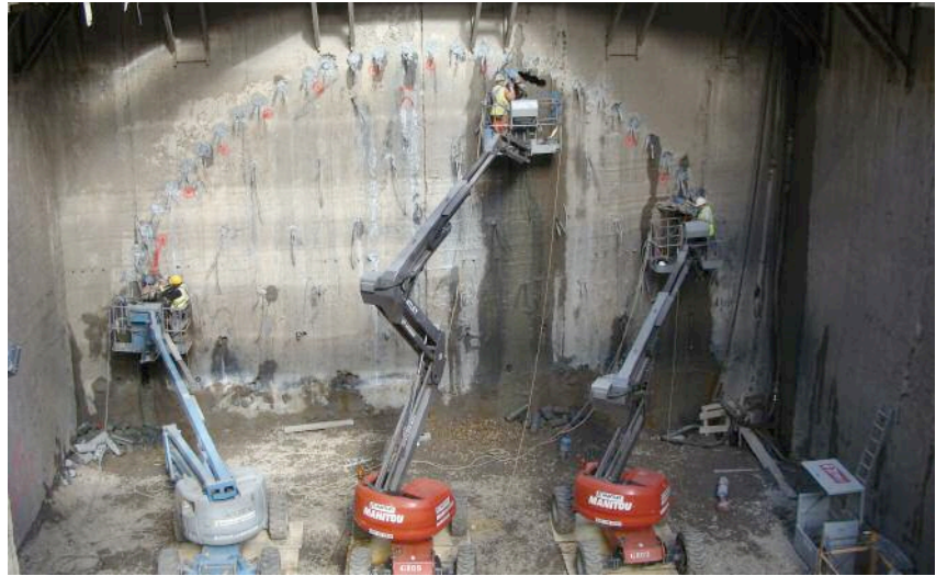
Above left: Special RMD Kwikform formwork installed in cut-and-cover Above right: Breaking through a wall in the SCL section
