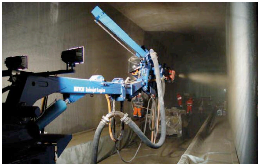
Above: A Meyco Logica 15 automatic spray robot applying a Fireshield membrane
