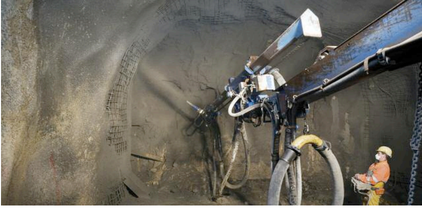
Above: Spraying polymer-modified concrete onto a tunnel wall in the Stetten salt mine to stabilise the tunnel and prevent water leakage. Right: Figure 1 – Relative rebound v concentration of polymer (data from Hagerbach gallery tests, Switzerland)
