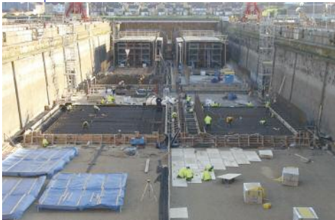
Above left: Special RMD Kwikform formwork installed in cut-and-cover Above right: Breaking through a wall in the SCL section
