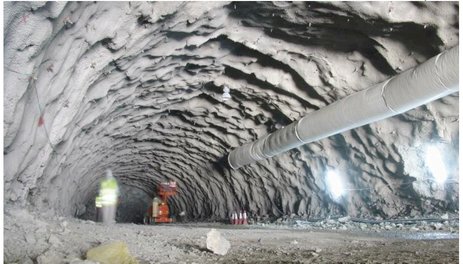
Above: Excavation within the NATM was co-ordinated in two stages
