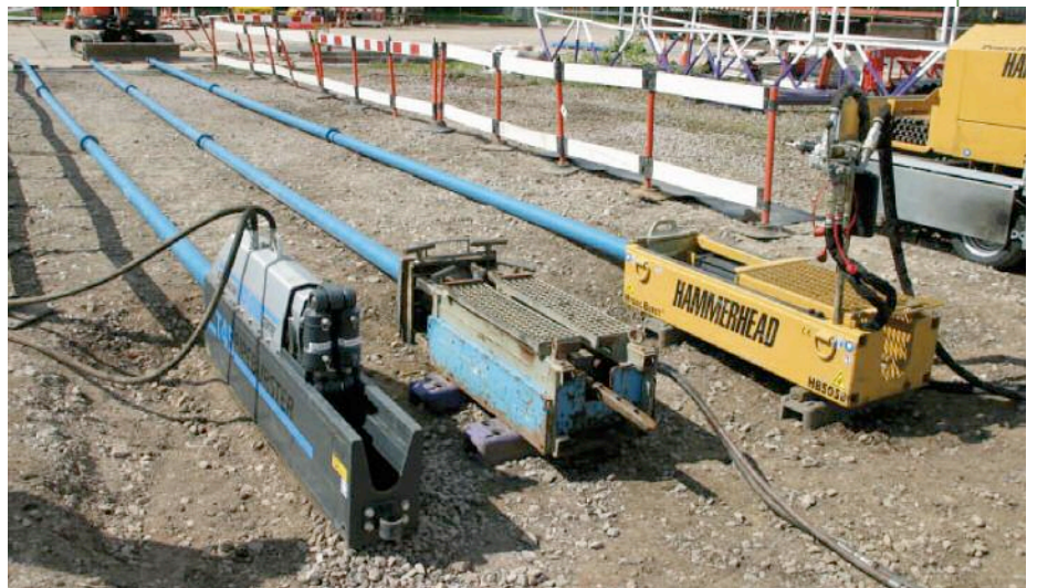
Above: The three pipe-bursting rigs on test laid out in parallel
