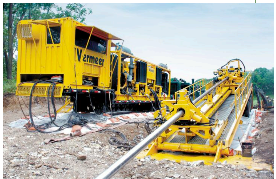
Below: The D1000x900 Navigator is Vermeer's largest HDD rig
