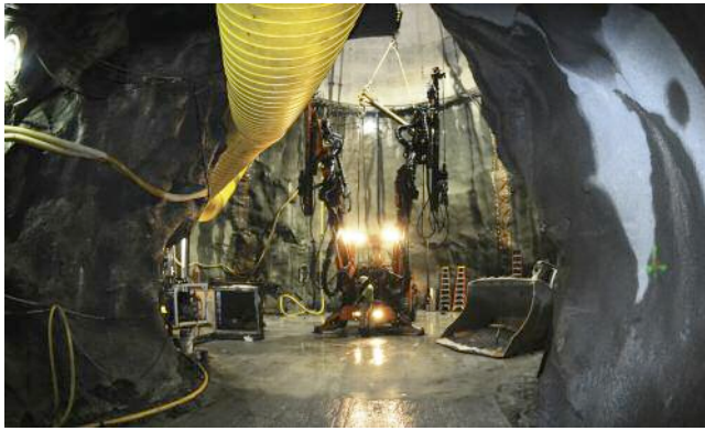
Above: In the South Cobb Shaft (TBM exit shaft), Shea/Traylor drove a 600ft drill & blast tunnel for the Influent Pump Station connection Above right: At the end of the 400ft Starter Tunnel, Shea/Traylor used forms and shotcrete to build 'gripper walls' for the TBM launch Below Left: The 27ft dia Herrenknecht TBM enters the 'gripper section' of the starter tunnel. The TBM was moved via a Barnhart Rail system up to the point where the grippers could take over
