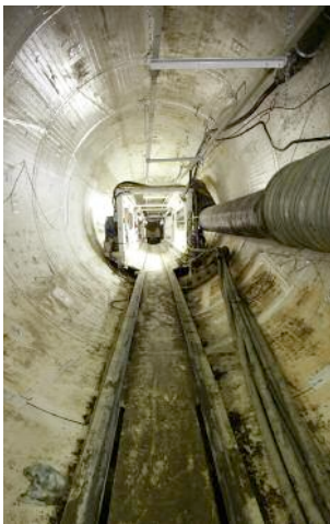
The novel PVC coated precast segmental lining used in Sacramento
