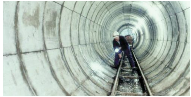
Above: Wedge block liner
