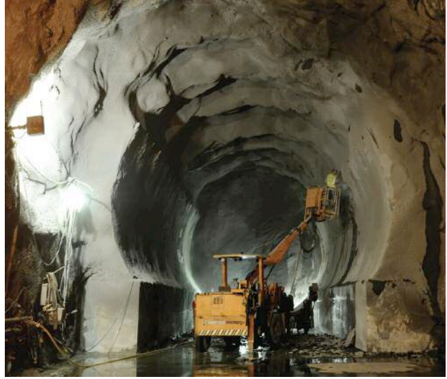
Above: In the South Cobb Shaft (TBM exit shaft), Shea/Traylor drove a 600ft drill & blast tunnel for the Influent Pump Station connection Above right: At the end of the 400ft Starter Tunnel, Shea/Traylor used forms and shotcrete to build 'gripper walls' for the TBM launch Below Left: The 27ft dia Herrenknecht TBM enters the 'gripper section' of the starter tunnel. The TBM was moved via a Barnhart Rail system up to the point where the grippers could take over
