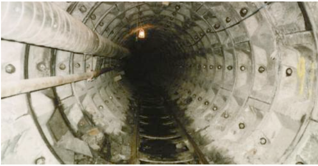
Above: Standard bolted segmental liner
