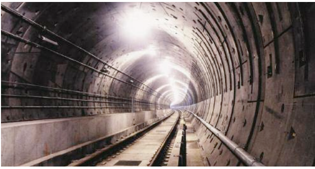
Left top: Tapered ring on the Sheppard Subway, Toronto Left bottom: Tapered precast liner design – Edmonton SLRT
