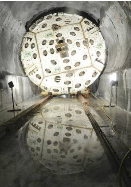
Above: In the South Cobb Shaft (TBM exit shaft), Shea/Traylor drove a 600ft drill & blast tunnel for the Influent Pump Station connection Above right: At the end of the 400ft Starter Tunnel, Shea/Traylor used forms and shotcrete to build 'gripper walls' for the TBM launch Below Left: The 27ft dia Herrenknecht TBM enters the 'gripper section' of the starter tunnel. The TBM was moved via a Barnhart Rail system up to the point where the grippers could take over
