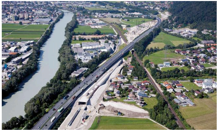
Above: The complex road, rail, stream and tunnel crossing at Stans
