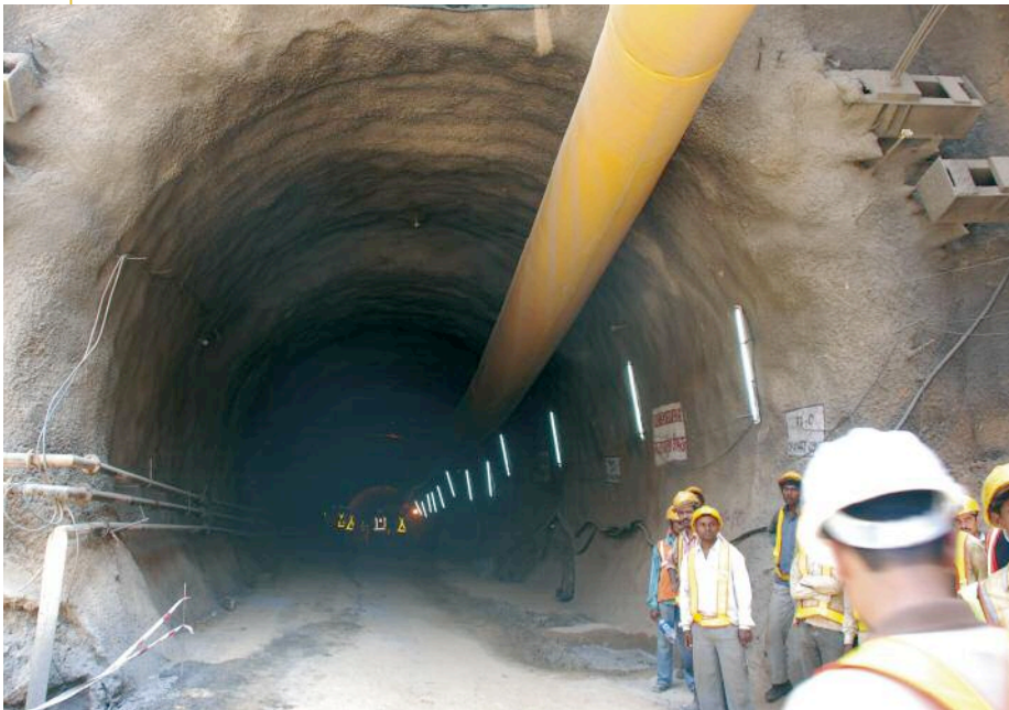
Above left: A view down the NATM section of tunnel south of Saket Station Above right: A typical cross section in a NATM tunnel section Left: This was the first NATM excavation in soft ground ever attempted by DMRC
