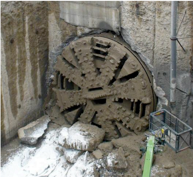
Above left: Breakthrough of an 8.16-m Wirth EPB TBM equipped with TunnelTec tools on the Castellanza metro project, Italy. The cutterhead is equipped with both static rippers and scrapers and disc cutters with carbide bullet inserts. Right: Disc cutters shown on the cutterhead of a 9.90m-diameter NFM Technologies TBM on completion of 1140m in a single month for the Madrid-Gijón high-speed railway route
