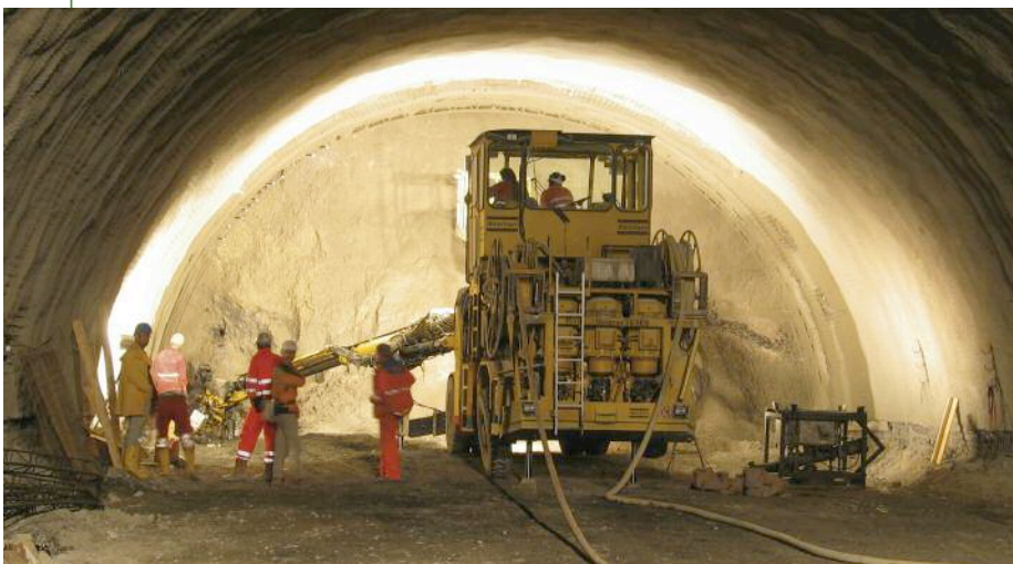
Left: Drill and blast on the longer tunnel section from Stans to Terfens village
