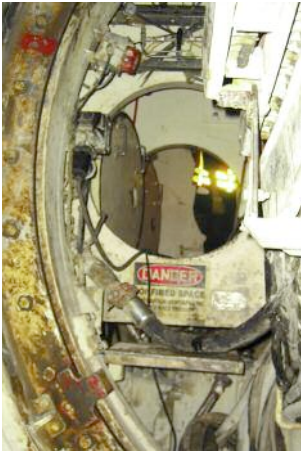
Left: A lack of space within JCT's Lovat EPBM results in extremely confined airlocks and face access
