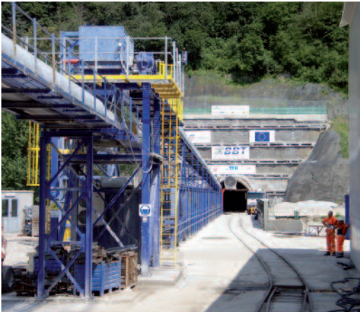
The belt storage at the Aica/ Aicha-Mules/ Mauls tunnel portal.
