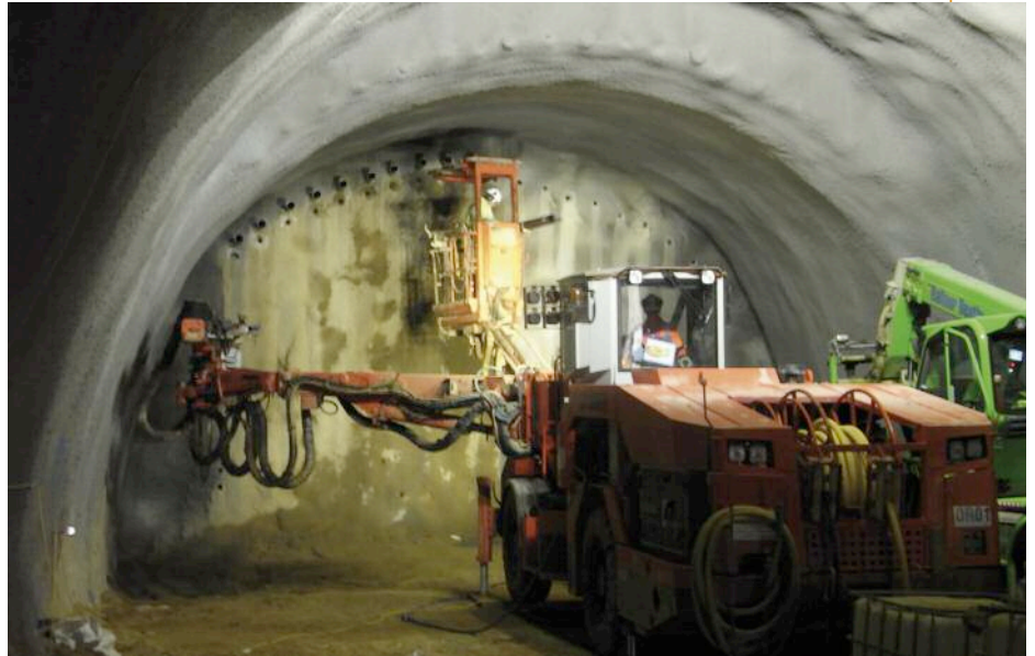
Above: Steel pipe canopy installation at weakest south end of bores
