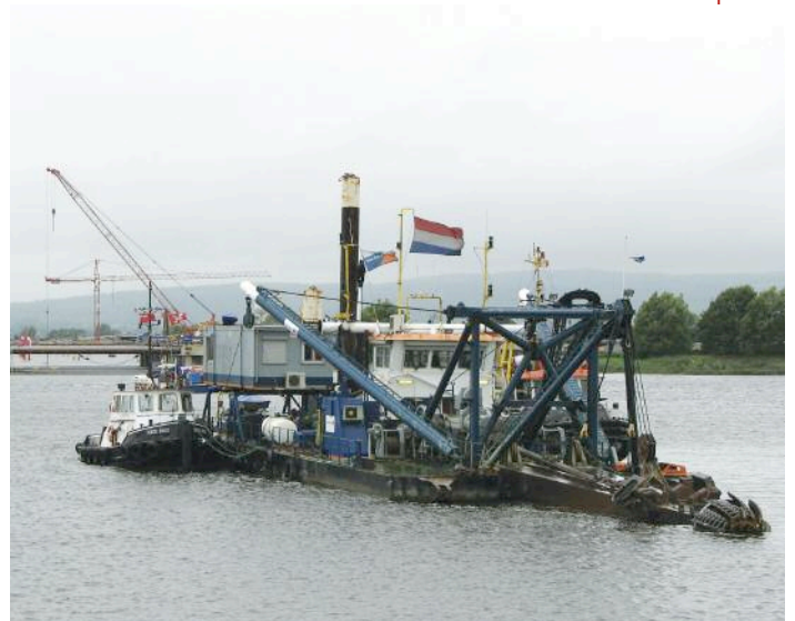
A suction-cutter will be used as shown on the Limerick Tunnel
