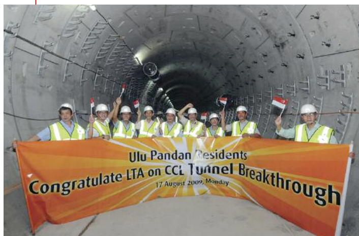
A view down the 33.3km long Circle Line
