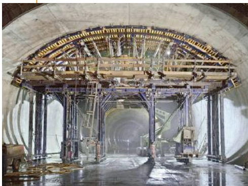
Above: The Doka formwork used for the Adelrain Fork section of the Lötschberg Tunnel at Frutigen by SATCO
