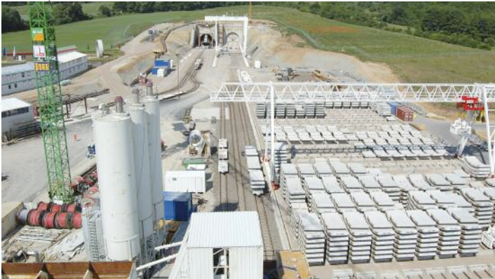
Above: The Finne Tunnel segment yard and portal
