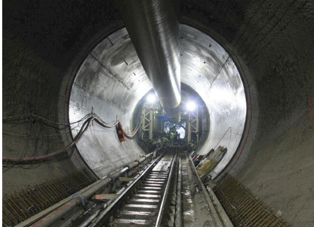
Above: Between the primary and secondary lining
