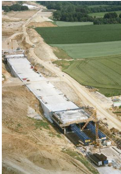
Above: Doka formwork being used on the Steinhaus Tunnel
