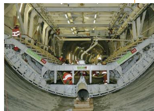
Above: Ceresola's invert shuttering currently being used in the Zurich Weinberg Tunnel for SBB
