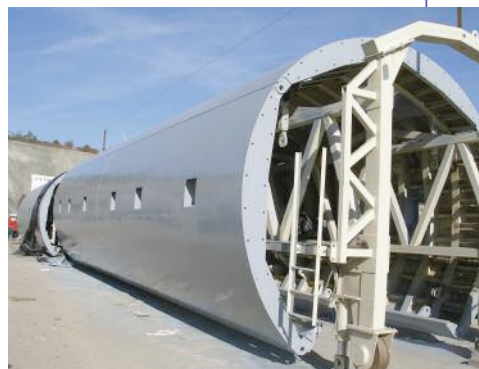
Above: The formwork for the final lining
