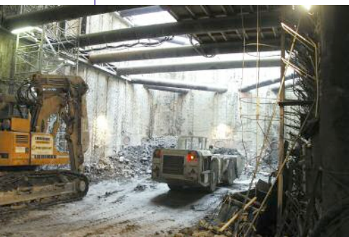
Above: Open cut station construction works underway at Bocskai road station and Keleti main railway terminus
