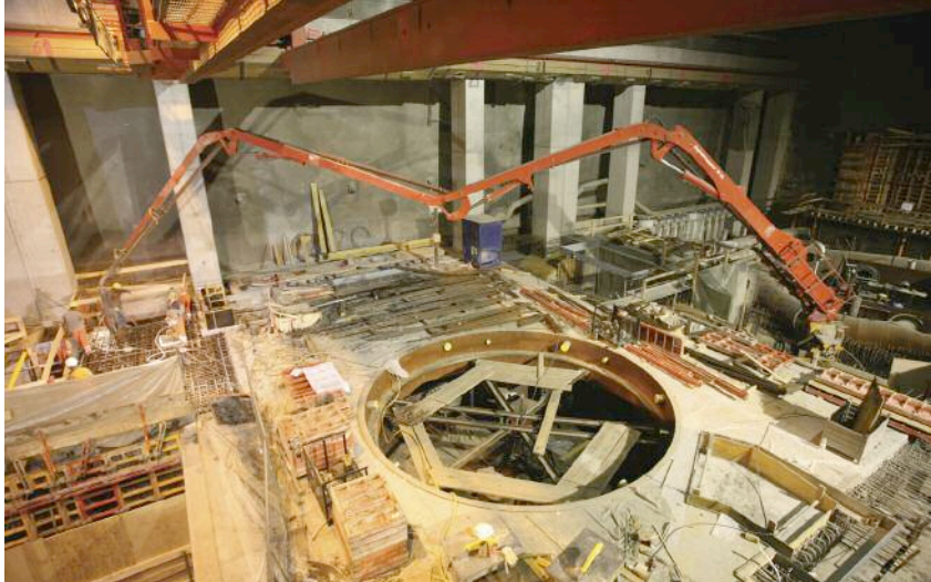
Left: Multiple concrete placement tasks were carried out in the underground Kopps II power station using a Putzmeister stationary boom MX 284 with a 'Z'-fold system and fed alternately by two columns.
