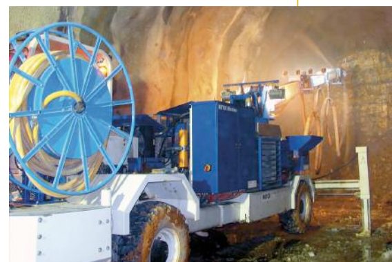
Below: At the shotcreted face of the Changuinola 75 HEP headrace tunnel
