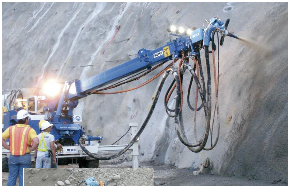
Above and left: Stabilising slopes on the Changuinola 75 hydroelectric project with a MEYCO Potenza Maxima concrete spraying rig
