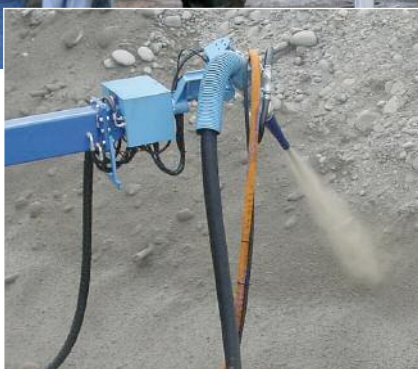
Above and left: Stabilising slopes on the Changuinola 75 hydroelectric project with a MEYCO Potenza Maxima concrete spraying rig
