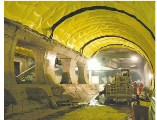
Above: Budapest's Line 4 Metro works
