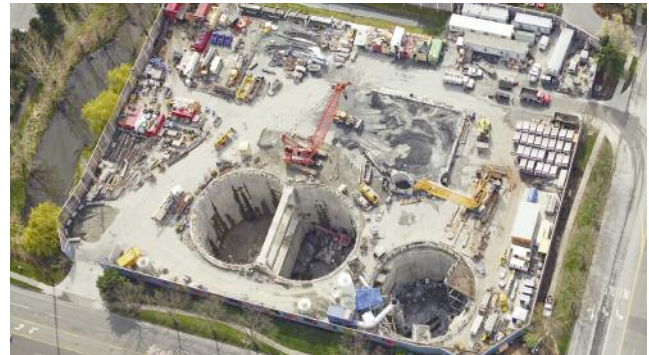
Top left: View of the East Tunnel; Above: The North Creek site, with the twin-celled IPS Shaft to the left and influent/portal shaft on the right; Left: KST's breakthrough on BT1 in early-November
