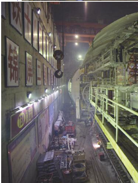
Above: The 12.43m diameter Robbins TBM began boring in mid-October 2008 Left: Robbins designed the back-up system with a steel shield to deflect heavy water inflows
