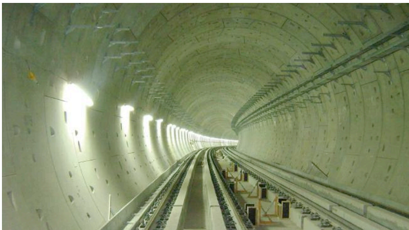
Above: A finished section of the metro tunnel
