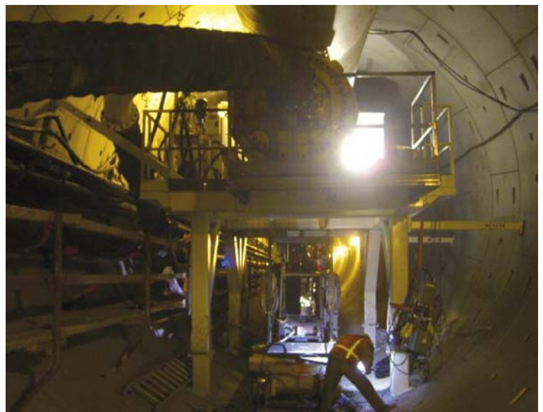
Right: A custom made platform supports one of the project's 20t Warman booster pumps
