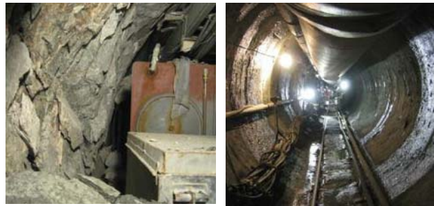
Clockwise from right: Seymour Capilano photos showing "stable" rock conditions; "fractured" rock conditions; and the "hazardous" conditions that caused Bilfinger Berger to halt the TBM drives
