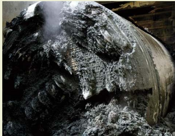
Above: Completion of the record-breaking 3055ft drive
