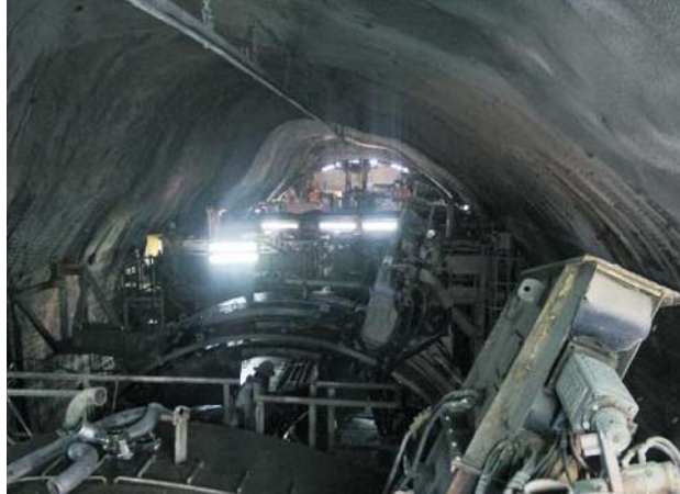
Above: View towards the face from the L2 area, showing overbreak
