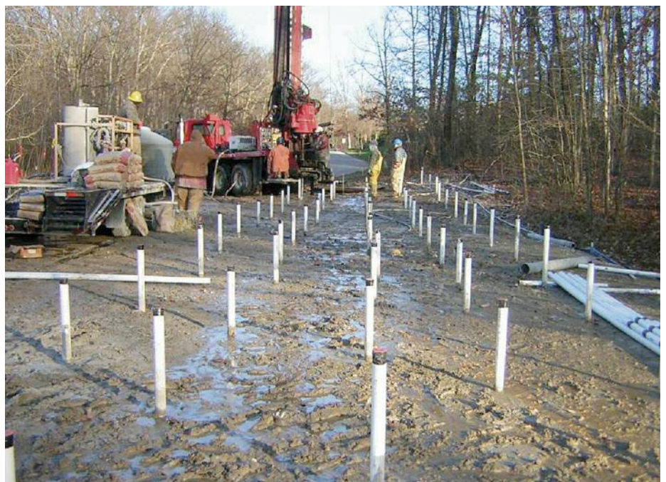
Above: Sleeve pipe installation (five rows) above a future tunnel trajectory in Columbus, Ohio, in 2008
