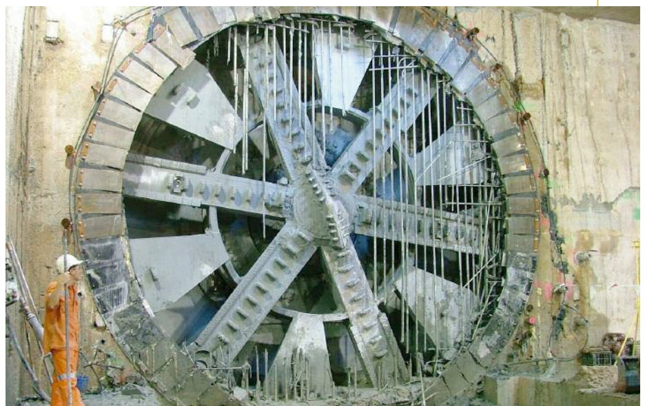
Below: Breakthrough on Perth's Metro Rail Project
