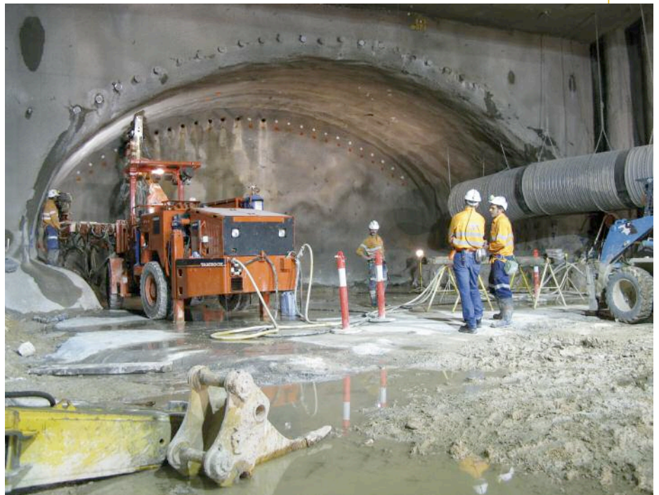
Above: Alwag canopy tube installation using the Tamrock Boomer
