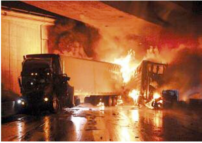
Above: Uncontrollable fire in the Santa Clarita Tunnel, on California's I-5
