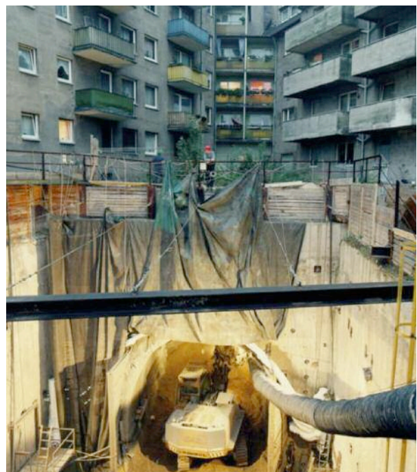
Above: Access shaft of the tunnel track in Düsseldorf
