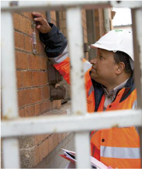
Above: Measuring possible settlement at the Jail
