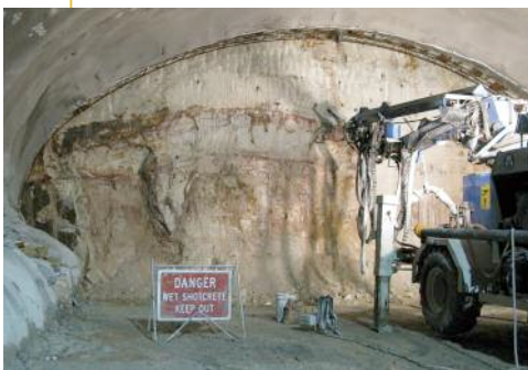
Above: The Meyco Suprema preparing to spray a lattice girder
