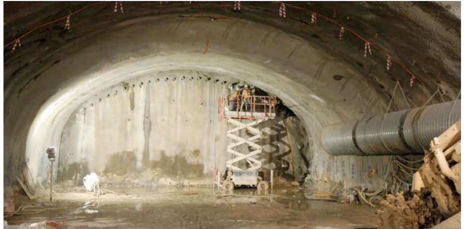
Above: Canopy installation on Brisbane's Boggo Road Tunnel
