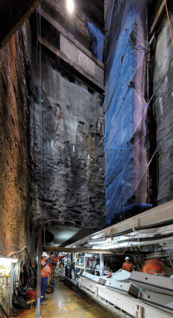
Above: View up the shaft on Sydney's City West Cable Tunnel
