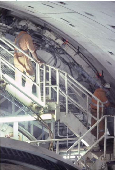
Above: One of the Herrenknecht TBMs Left: Segment erection underway using the TBMs automated erector machine
