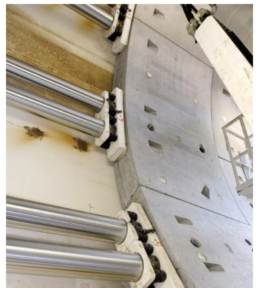
Right, and above: Rings had flat-faced edges. The joints helped to ease segment removal at cross passages, where special segments also formed 'diamond dowels' for stress distribution and so avoid the needs for framing
