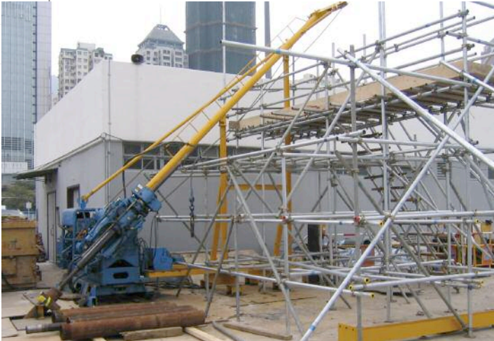
Above: Drill site and drill rig set up
