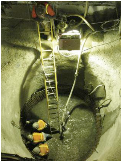
Above: Sump excavation at cross passage 5 fighting water inflows
