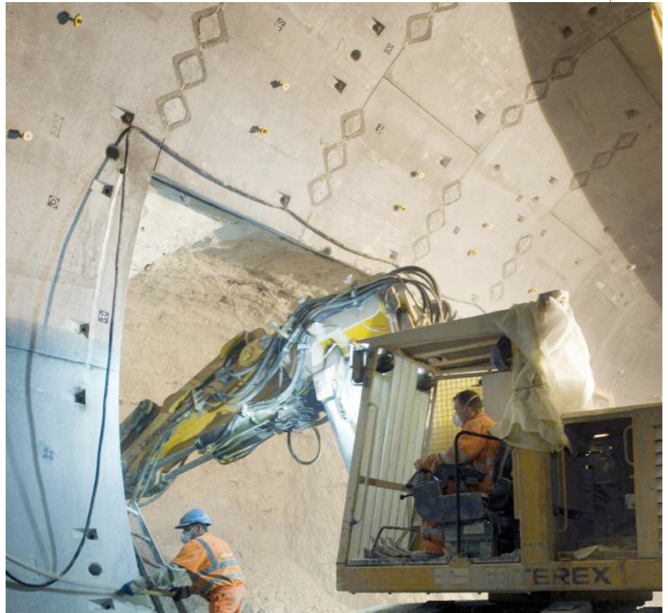
Right, and above: Rings had flat-faced edges. The joints helped to ease segment removal at cross passages, where special segments also formed 'diamond dowels' for stress distribution and so avoid the needs for framing
