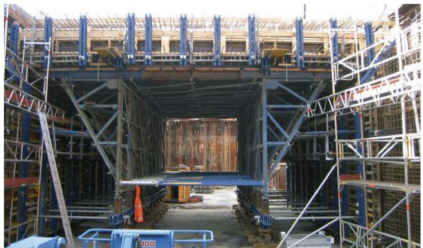
Right: Doka's travelling formwork units at work in Trondheim, Norway
