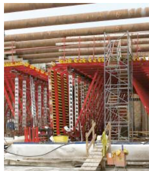
Above: Concreting works underway for the immersed tube tunnel near Limerick, Ireland, to cross the river Shannon
