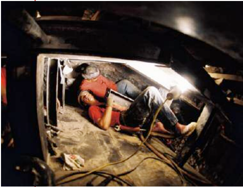
Above: Pic 4 – Hand mining over the shield
