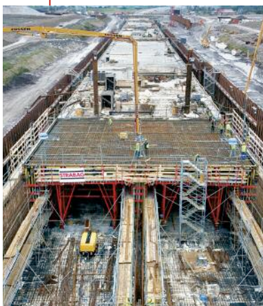
Above: Concreting works underway for the immersed tube tunnel near Limerick, Ireland, to cross the river Shannon
