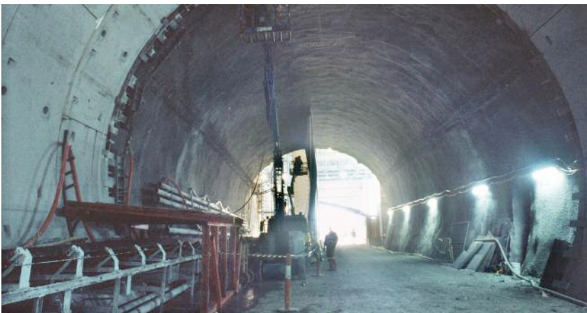
Below: Lining works at one of the tunnel portals
