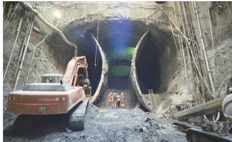
Above: Centre bench excavation of a Concourse Cross Adit (CCA)
