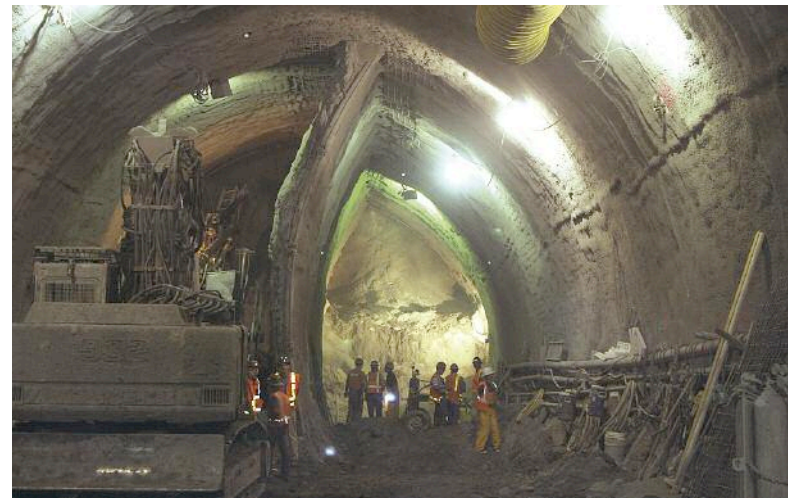
Above: SEM excavation of a Beacon Hill Station platform tunnel
