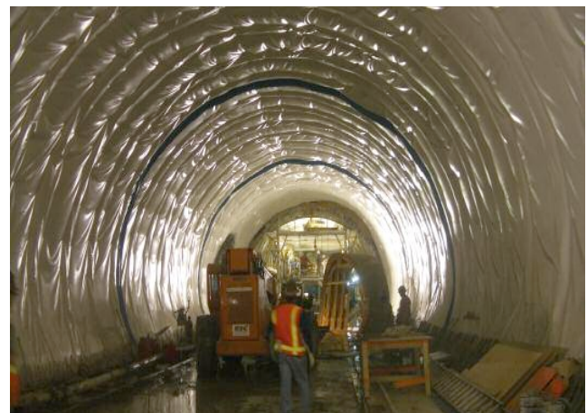
Below: Waterproofing of the Platform Tunnels
