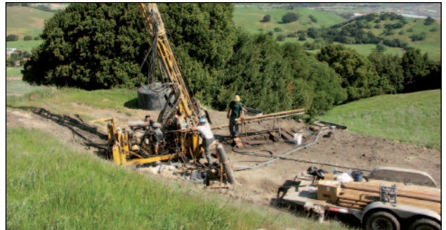
Geotechnical Drilling for Tunnel Investigation
