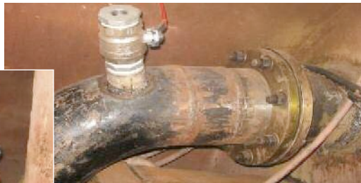
Below and right: The balancing pipes in the TBM – for flushing provision
