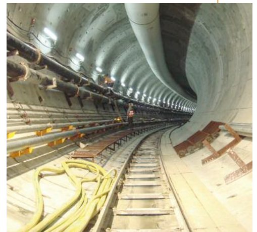
Right: Finished tunnel lining
