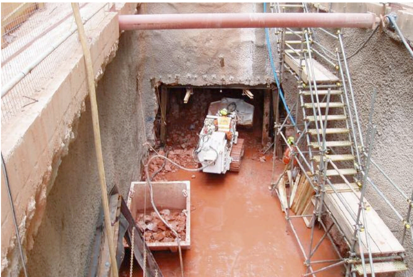
Below: The project shaft with muck out in progress
