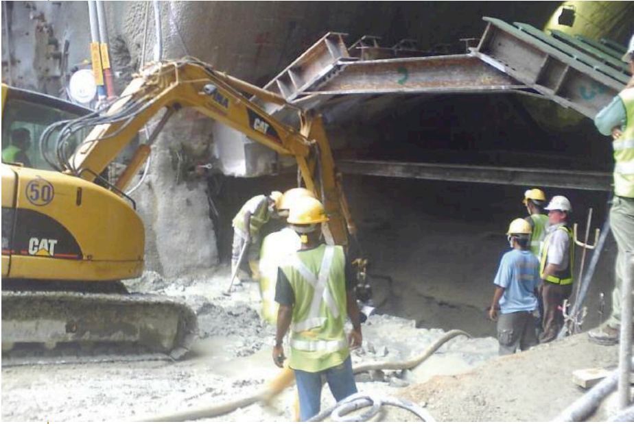
Left and Above: Improved accessibility of machinery made possible by the A-frame installation
