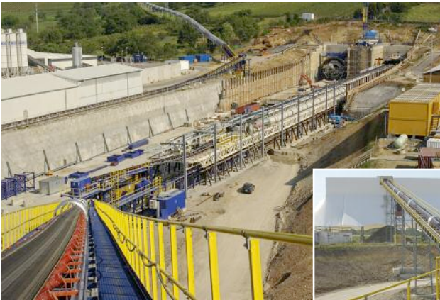
Left and below: Katzenberg's portal area, showing the installation of the Marti Technik conveyor system and temporary muck storage
