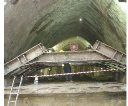
Left and Above: Improved accessibility of machinery made possible by the A-frame installation
