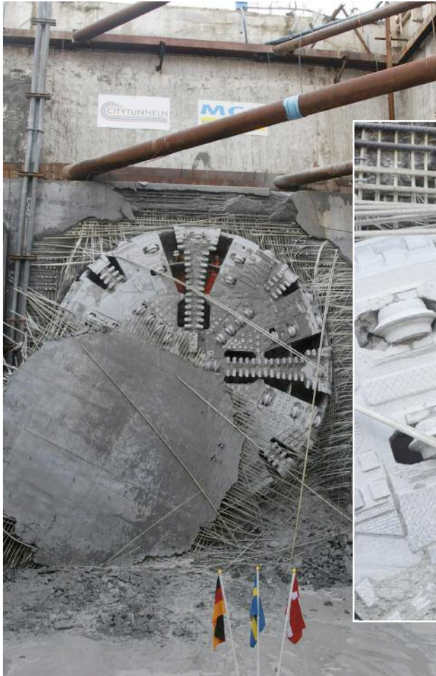
Final breakthrough of the first TBM on the twin rail tube drives in Malmö
