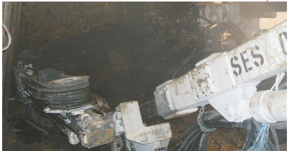
Above: The jumbo drill rig working at the face
