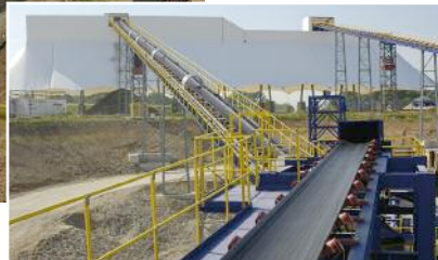
Left and below: Katzenberg's portal area, showing the installation of the Marti Technik conveyor system and temporary muck storage
