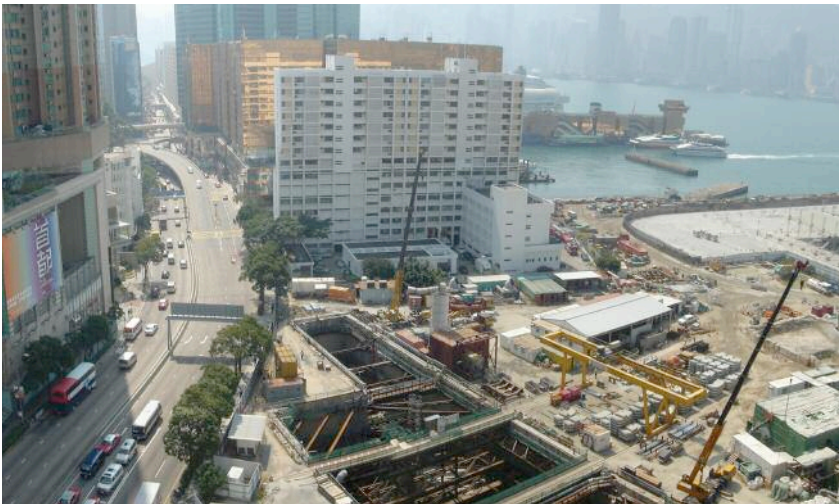
Left: The launch shaft in West Kowloon
