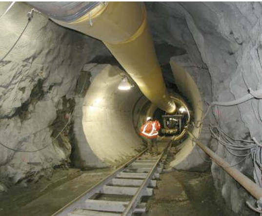
Above left: TBM launch zone at the face of the starter tunnel; Middle: Installing support through fault zone F1; Right: Modified 300° steel set supports without invert sections through fault F1 (above photos by D Brox)
