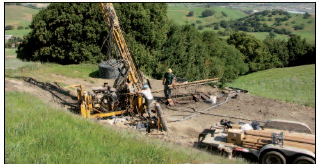
Geotechnical Drilling for Tunnel Investigation
