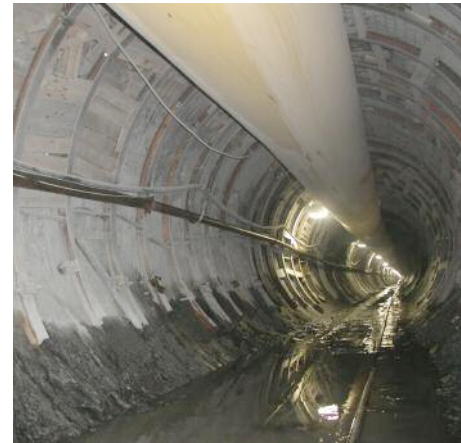
Above left: TBM launch zone at the face of the starter tunnel; Middle: Installing support through fault zone F1; Right: Modified 300° steel set supports without invert sections through fault F1 (above photos by D Brox)
