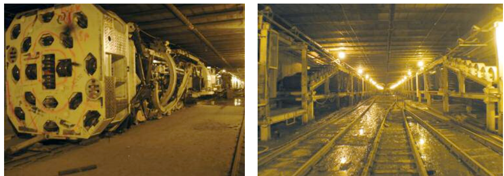
Below left: Walk of the partially assembled Robbins TBM through the immersed tube to the launch starter tunnel; Below right: Start of the twin TBM drives and headframes of the conveyors
