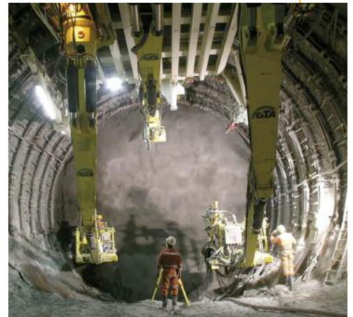
Above: Spraying the face on the Gotthard HSR Tunnel in Switzerland
