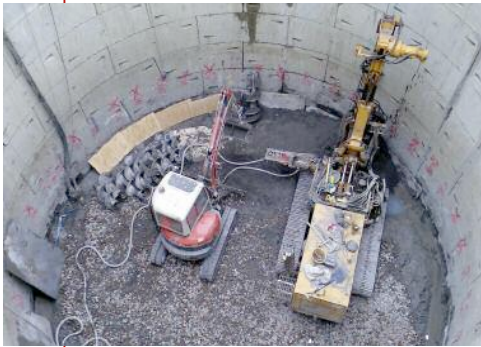
Above: Shaft construction well underway
