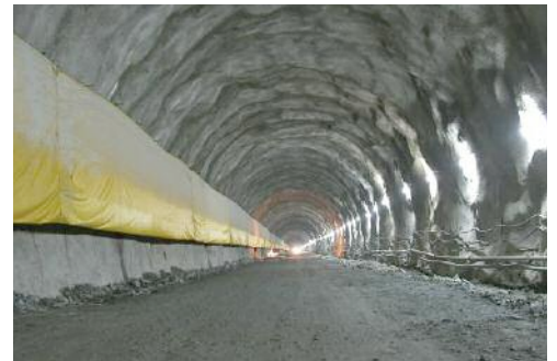
Above: The Kang Chon 1 Tunnel
