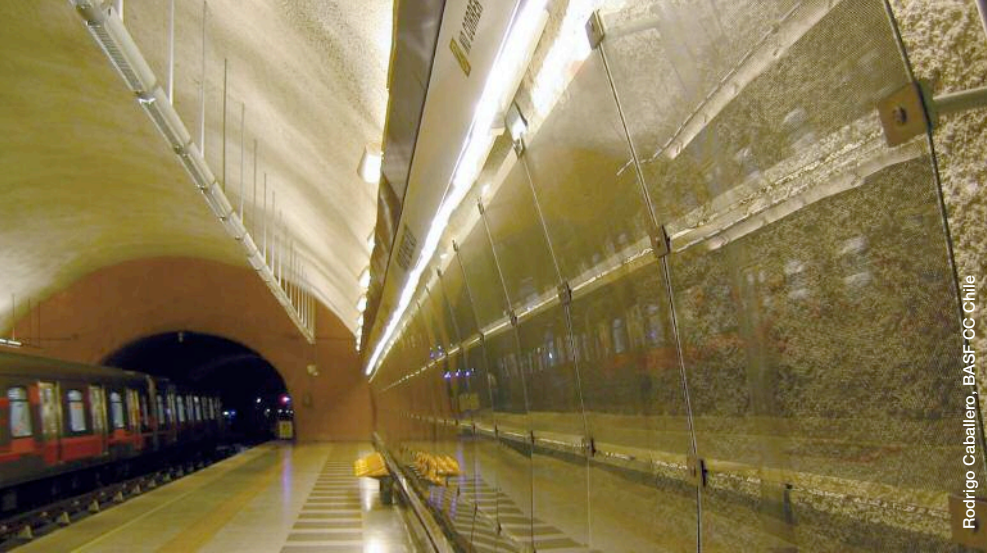
Above: Glass panels over rough sprayed concrete on Line 4 of the Santiago Metro
