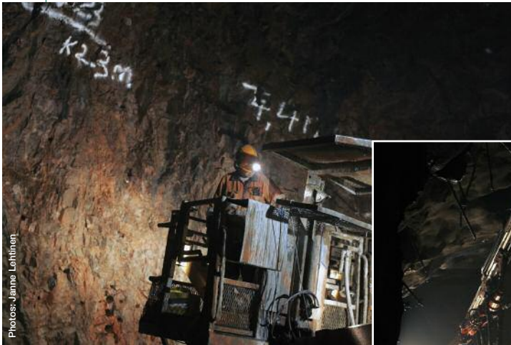
Left and below: Lemminkäinen's Sandvik Tamrock Axera T11 drill rig in use under the centre of the city
