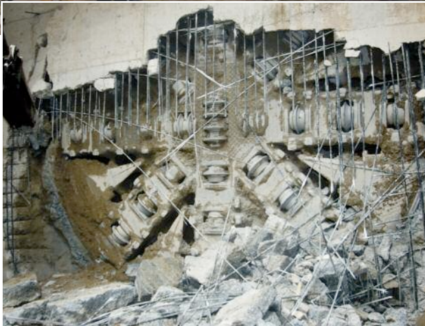
Second hole through at Botanical Gardens, Circle Line, Singapore
