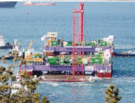
Float-out of first element of Busan-Geoje immersed tube
