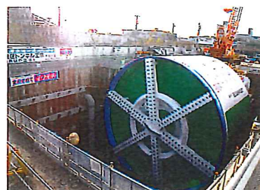
Photo 1 Before start on the surface (Machine setting completed)
