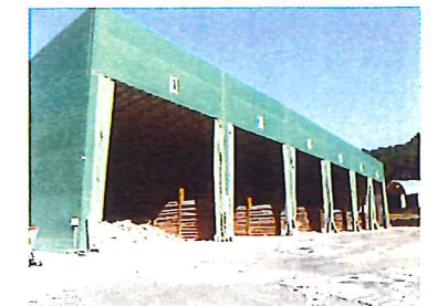
Photo 3 Large tent for storing excavated muck
