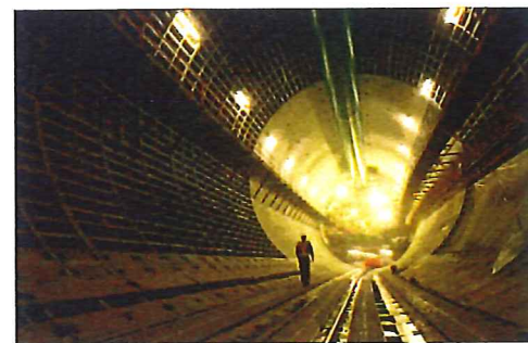
Photo 1 Shield tunnel (clockwise tunnel)
