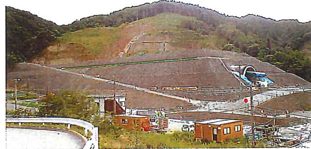
Photo 1. Protection embankment
