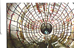
Photo 2 Completed entire facility
