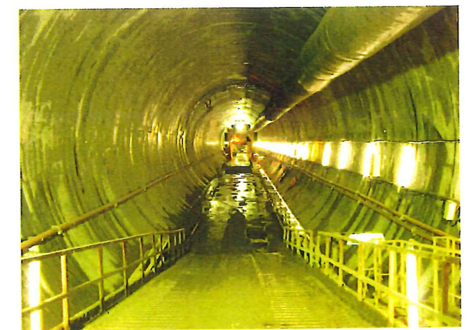
Photo 2 Completed primary lining
