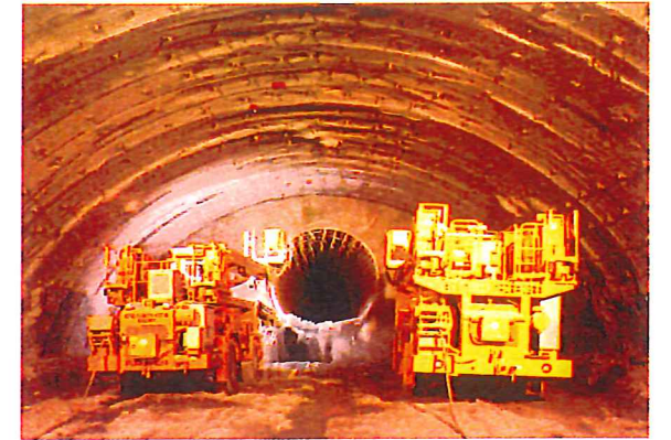
Photo 1 TBM drift with enlargement
