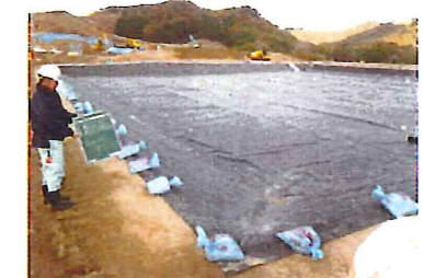
Photo 2 A layer of impermeable sheets
