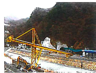
Photo 1 Belt conveyor outside the tunnel
