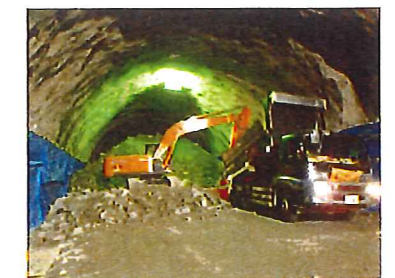
Photo 4 Temporary storage of excavated muck in the tunnel
