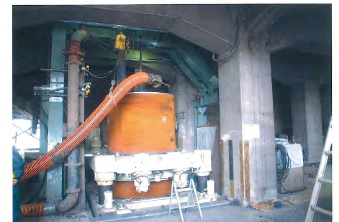
View of piling
