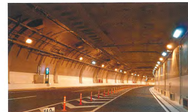
View of the completed cut-out work
