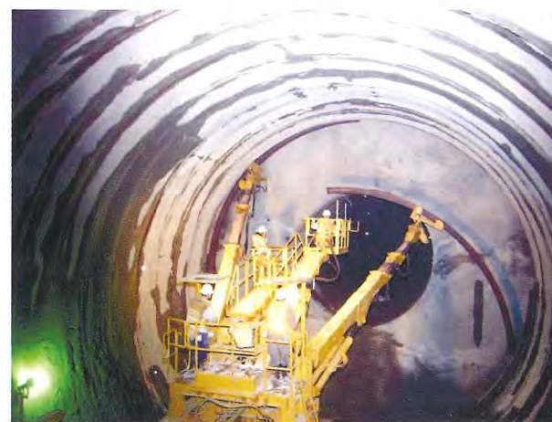
Construction of the main tunnel
