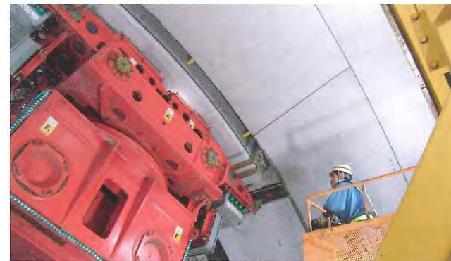
One-pass segment with smooth inner surface
