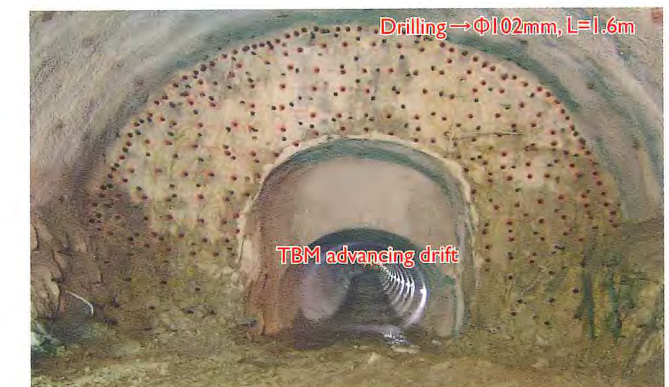
Drilling with rock breaker
