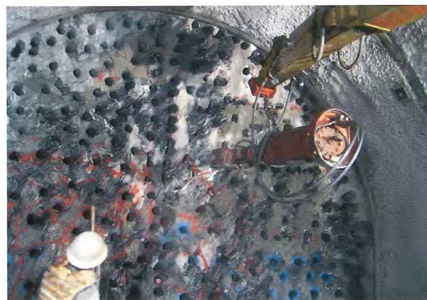
Driving with rock fracturing
