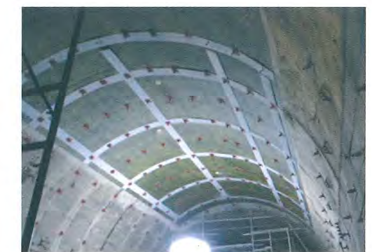
Photo 2 Restoration of the Daiichi Yoneyama Tunnel on the Shin-etsu Honsen railway
