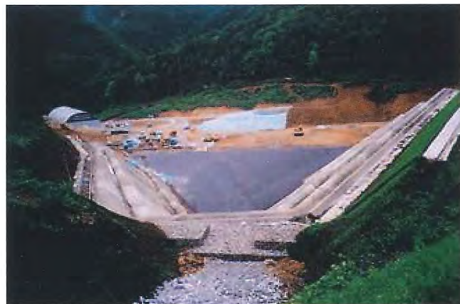
Impervious sheet placed at the bottom
