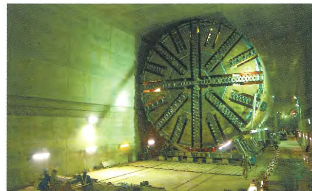
Horizontal movement of the shield machine
