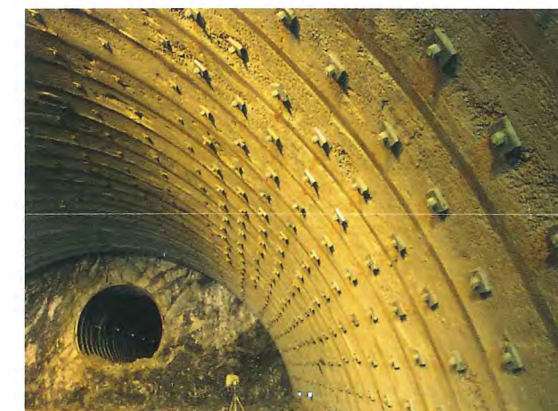
Driving the prestressing steel bar pattern
