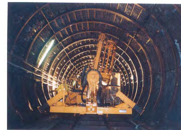
Driving the cable bolts from the TBM-bored drift
