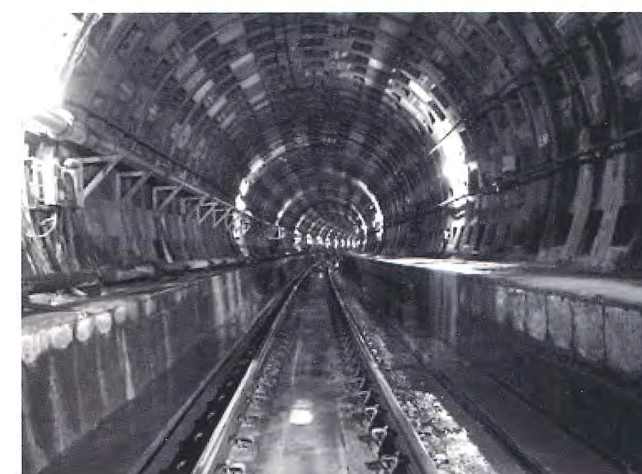
Before placement of the secondary lining
