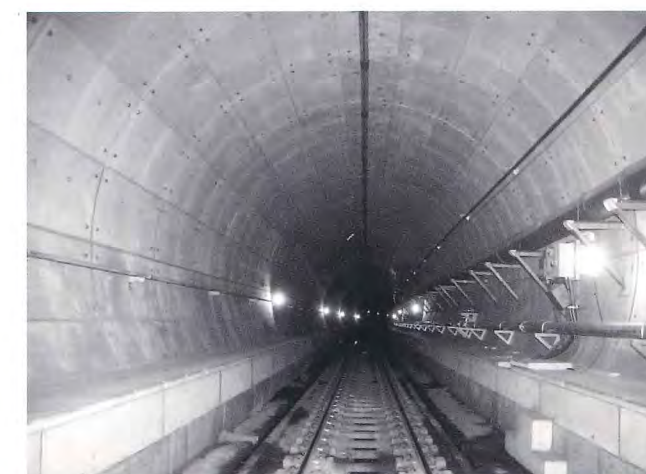
After placement of the secondary lining
