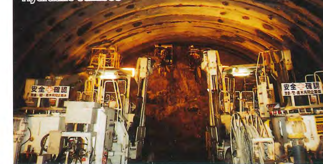
Main Tunnel Excavation by Two 2-boom Wheeled Hydraulic Jumbos
