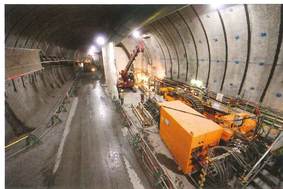
Photo 1 1,000 m-class ultra-long pilot boring
