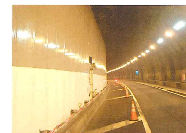
Photo 1 Placement of the protector (road side)
