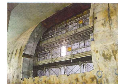
Photo 2 Segment cutting (work side)
