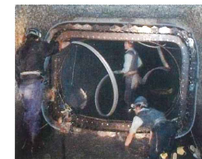
Photo 1 Reconstruction (in the pipe)
