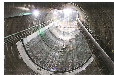
Photo 3 Lining in the WT section
