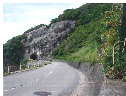
Photo 1 Shimoda Zuido before the construction
