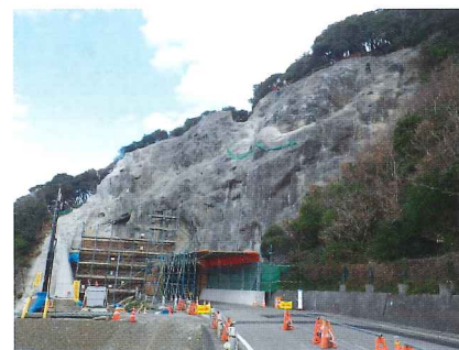
Photo 3 Safety measure on the slopes at the portal perimeter
