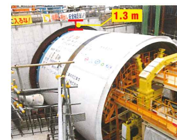
Photo 1 Ramp B starting area
