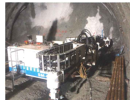
Photo 1 New drilling machine
