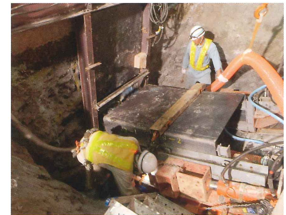
Photo 2 View of the box in place (placement of the steel box)
