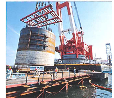
Photo 1 Placement of a caisson's cutter unit
