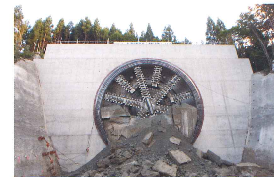
Photo 1 SENS's breakthrough to the portal
