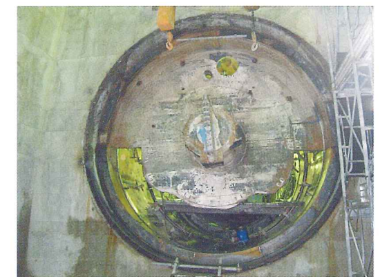
Photo 2 After dismantling of the face plate
