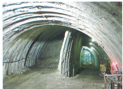
Photo 1 Central diaphragm (CD) method
