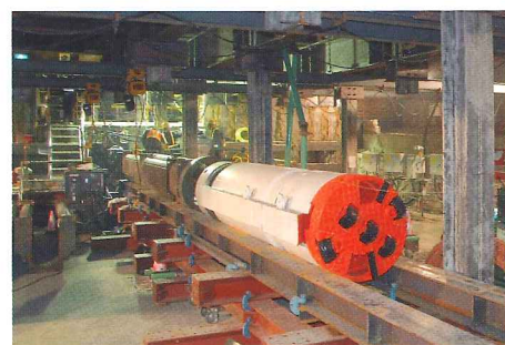
Photo 1 Pipe roof drilling machine
