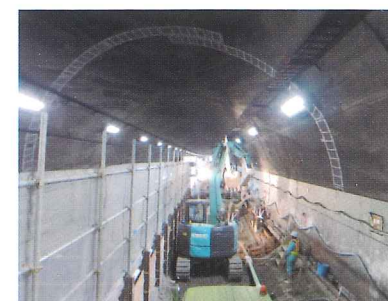
Photo 1 Repair of the left lane
