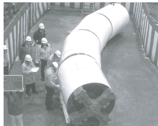
Photo 1 Main assembly of the excavator
