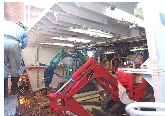
Photo 3 Open type shield machine
