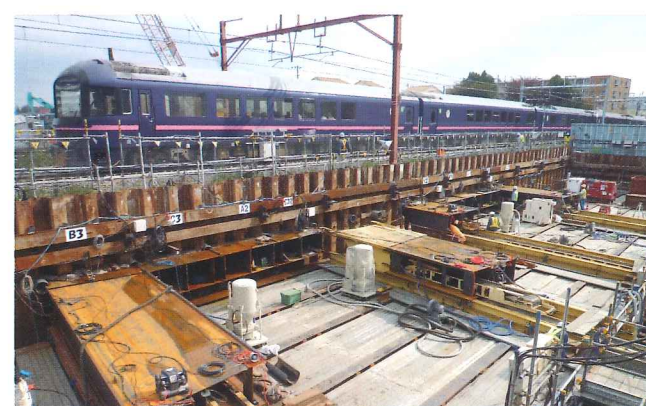
Fig. 3 Work in the starting shaft
