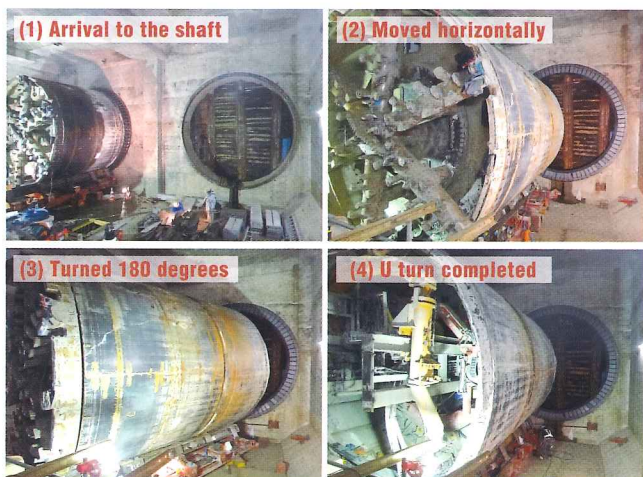
Photo 2 U turn process of the machine
