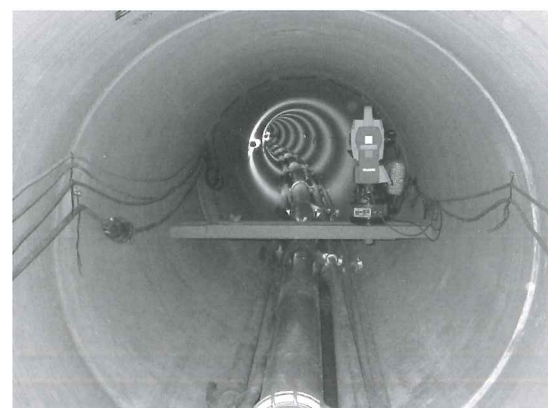
Photo 2 Installation of automatic survey equipment
