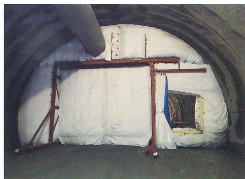
Fig. 1 Movable balloon bulkhead (view from the face side)
