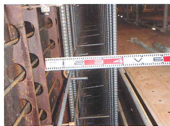
Fig. 5 Assembled PBL and side wall reinforcement
