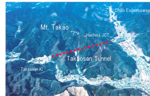
Photo 1 Overview of the Takaosan Tunnel
