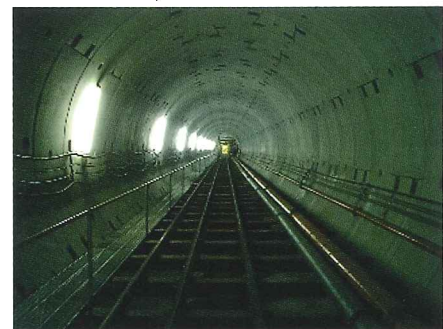
Photo 1 Inside the shield tunnel
