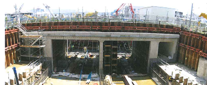
Photo 1 View of the construction site
