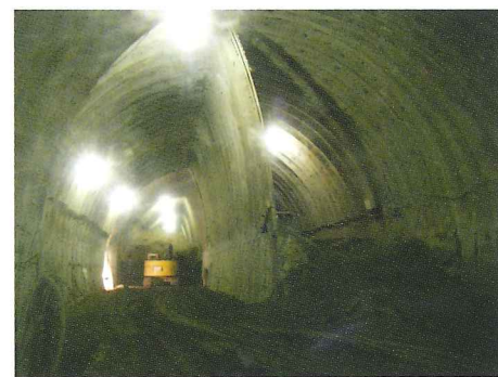
Photo 1 View of the large-section station tunnel under construction
