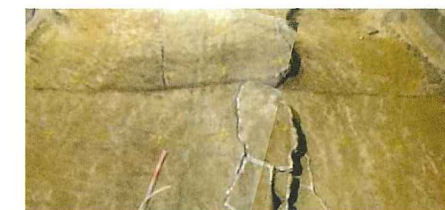
Photo 1 Damaged invert
