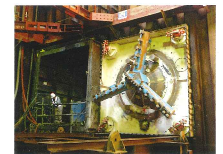
Photo 1 Breakthrough of the shield machine: B2
