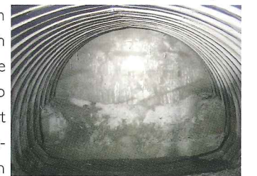
Photo 1 Early section closure
