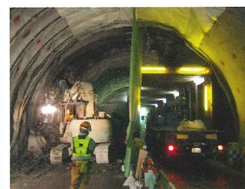
Photo 1 Excavation of the branching section
