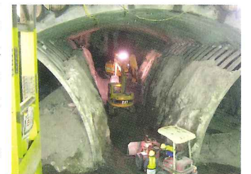
Photo 1 Upper half excavation
