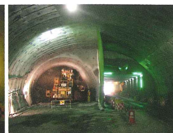
Photo 2 Excavation of the section close to the existing tunnel
