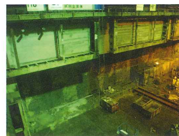
Photo 1 Tunnel shell structure
