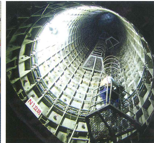
Photo 2 Completion of tunneling
