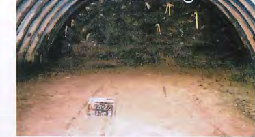
After Face Reinforcing
