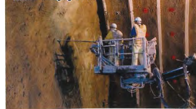
Remote Charging Work
